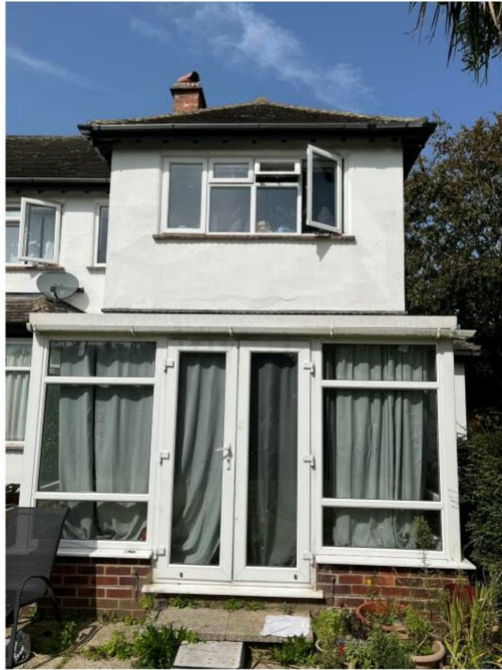
Existing Rear elevation Showing conservatory to be replaced
