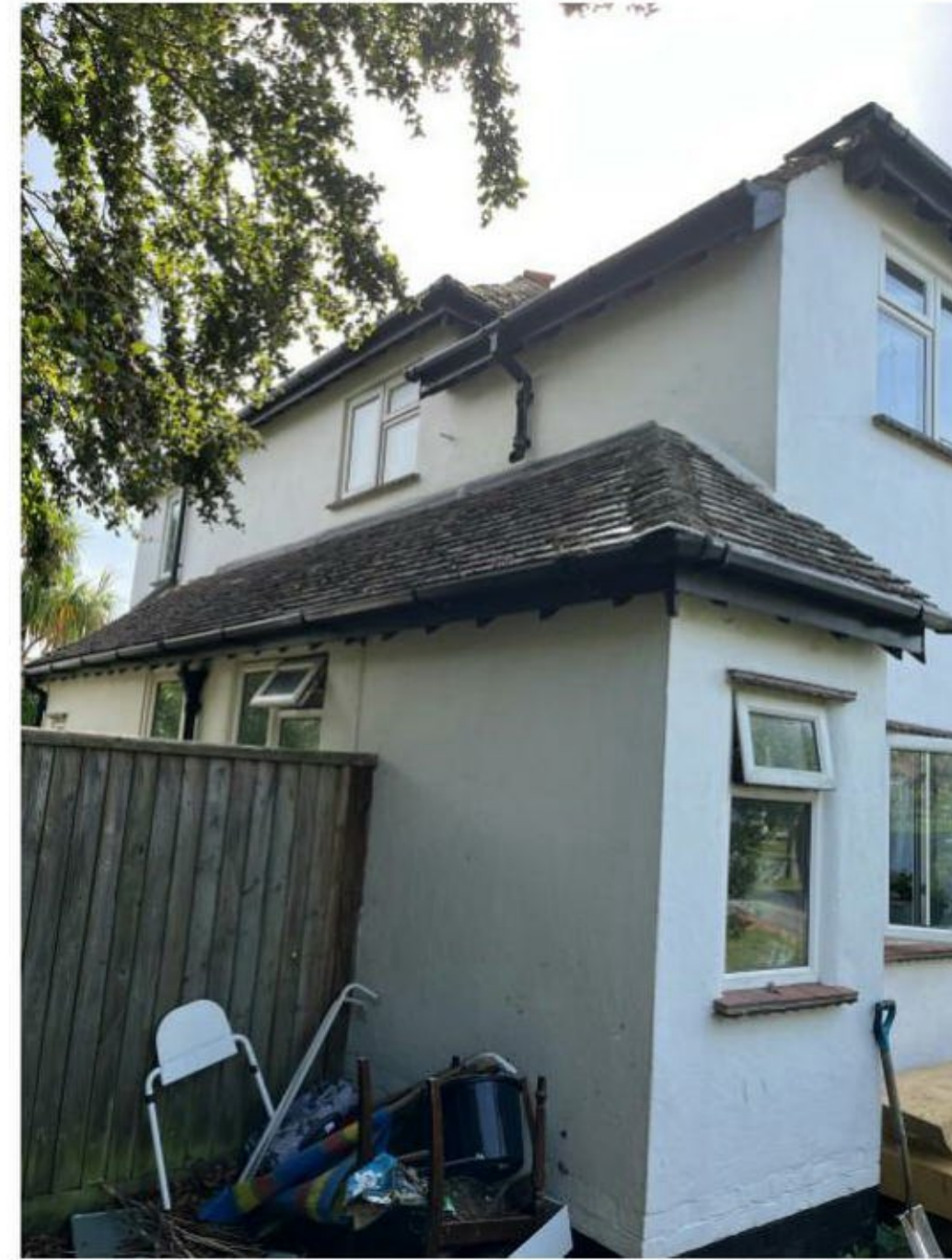
Existing Side Extension to be Thermally upgraded
