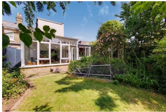
Rear elevation of property
