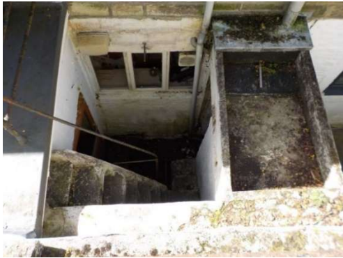
Rear lightwell of 8 Wood End
