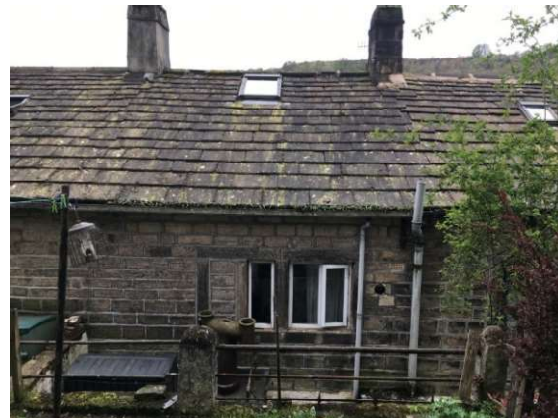
Rear elevation of 8 Wood End
