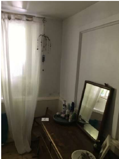
Stud partition wall separating bathroom from landing The wall would be moved 300mm further into the bathroom to widen the existing landing to accommodate the proposed new door
