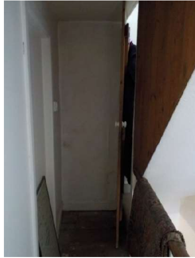
Proposed location for new door opening (internal) The proposed new door would open off the first-floor landing, which would be widened by moving the modern stud wall on the left
