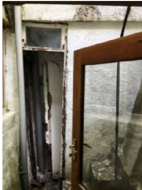
View of the outside toilet from the lightwell
