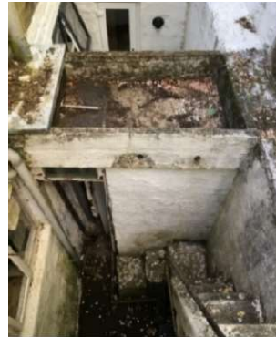
Redundant outside toilet from roof of offshot
