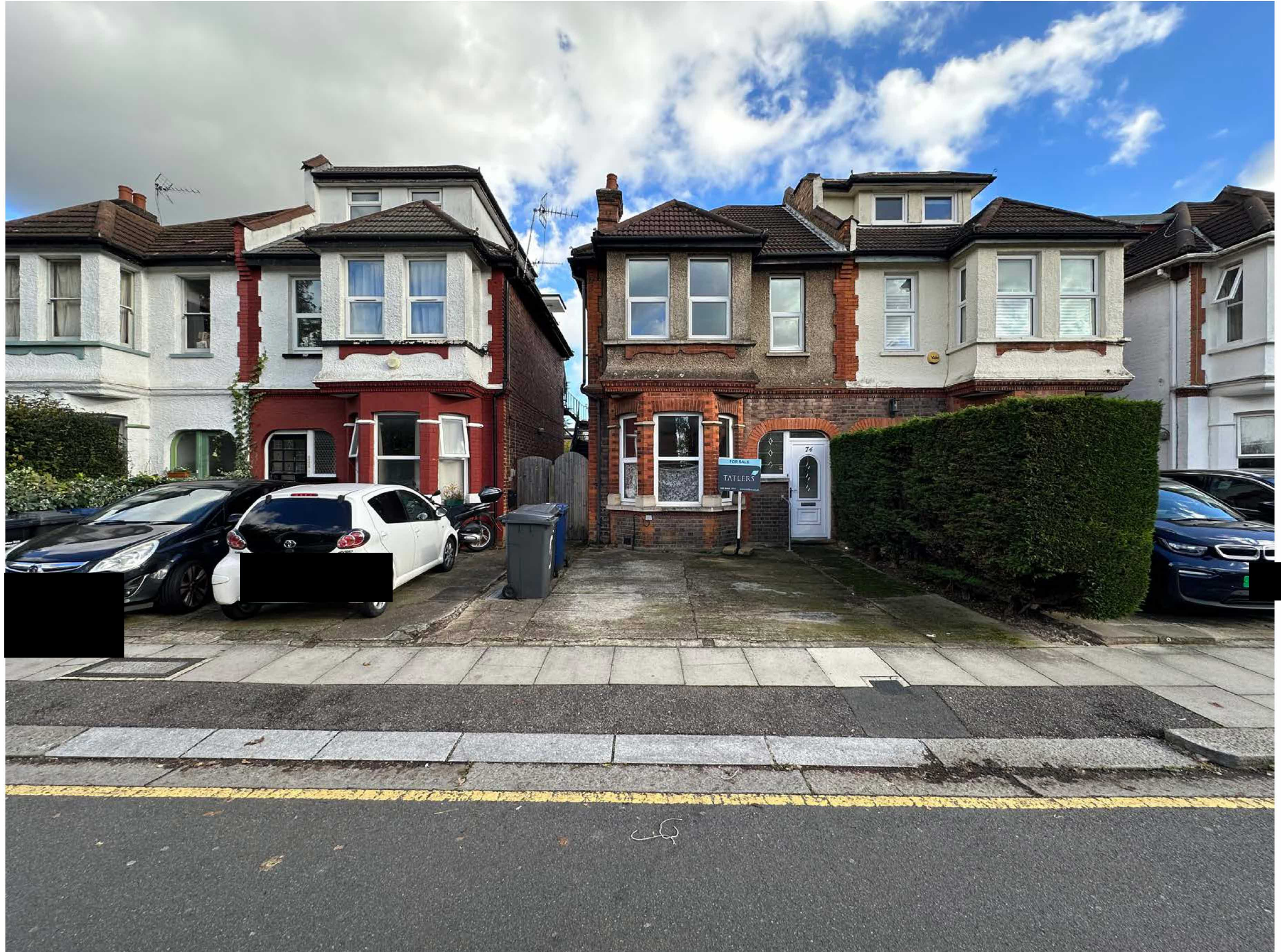
Figure 003 - View of front elevation
