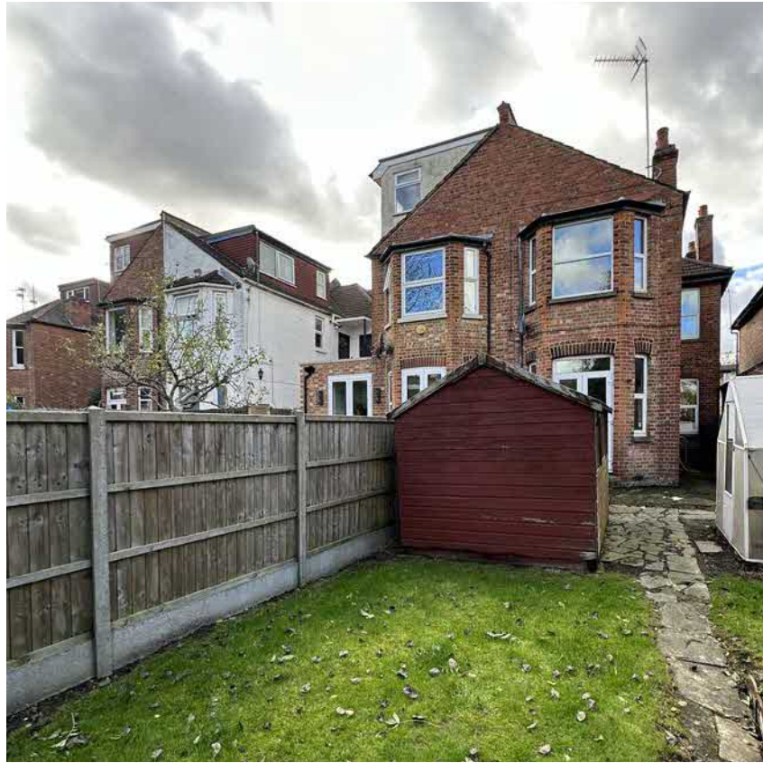
Figure 011 - View of rear elevation towards neighbouring property (No.72)
