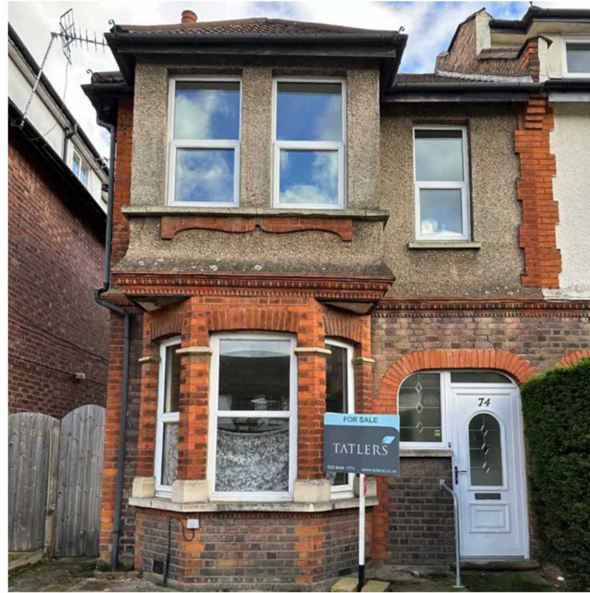
Figure 005 - View of front elevation
