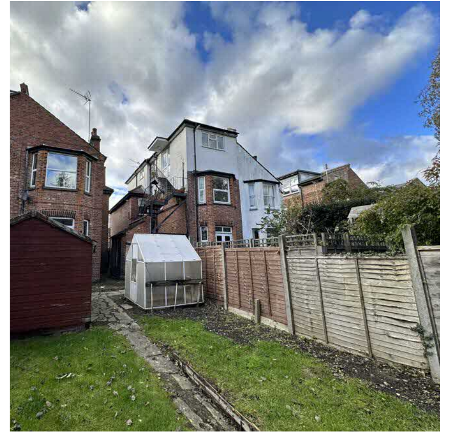
Figure 013 - View of rear elevation towards neighbouring property (No.76)
