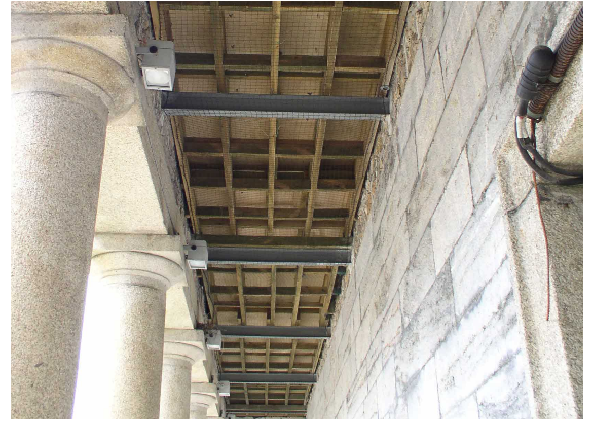
Fig. 5: View of the roof behind
