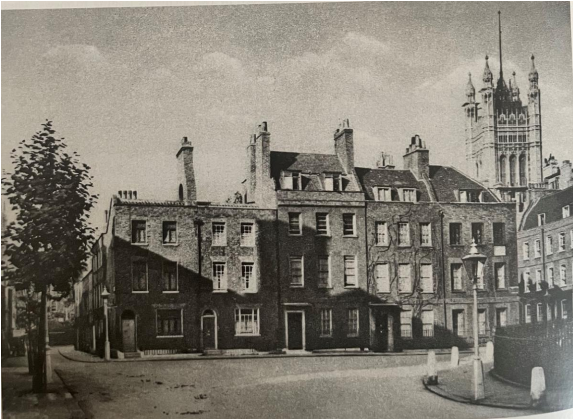
Figure 1 - The north side of Smith Square in 1926
