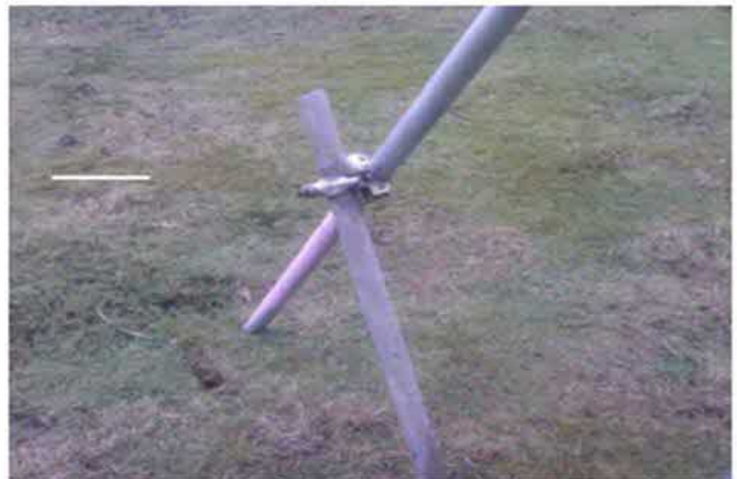
Typical Ground Anchor Method
