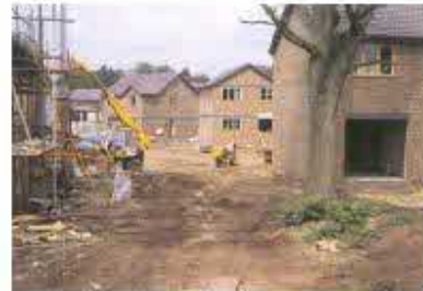
Ground protection is essential to maintain the health of tree roots on construction sites.
