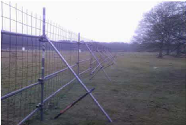
Typical Barrier Construction
