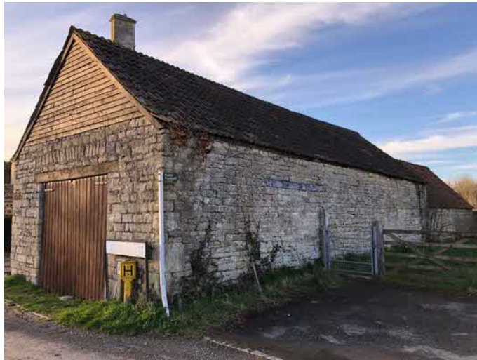
Photograph 2: Barn – south gable and east elevations (April 2018).
