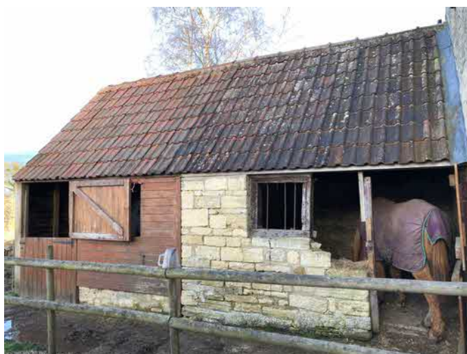
Photograph 3: Stable – west elevation (April 2018).
