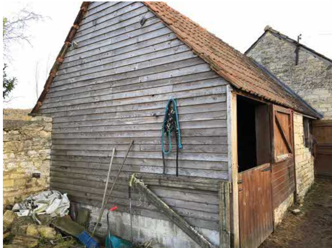
Photograph 4: Stable and Barn – north gables (April 2018).
