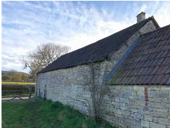
Photograph 5: Barn and Stable – east elevation (April 2018).
