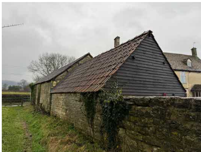
Photograph 4a: Stable and Barn – north gables (December 2023).
