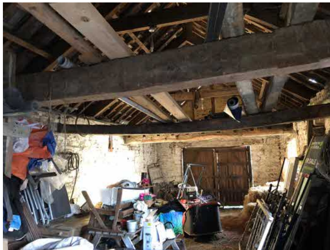
Photograph 8: Barn – interior (April 2018).
