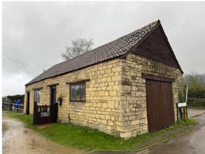
Photograph 1a: Barn – west elevation and south gable (December 2023).
