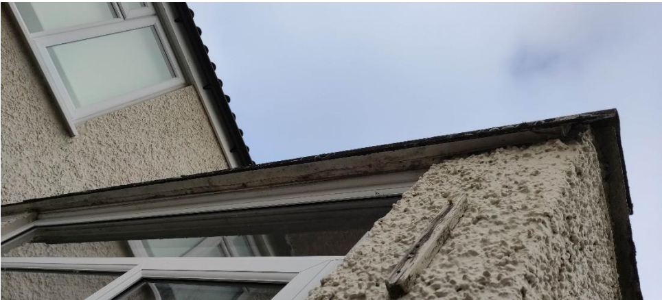
Fig.6 Detail view of the existing extension's ridge.
