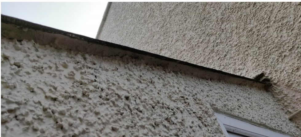
Fig.7 Detail view of the existing extension's roof edge (Front).
