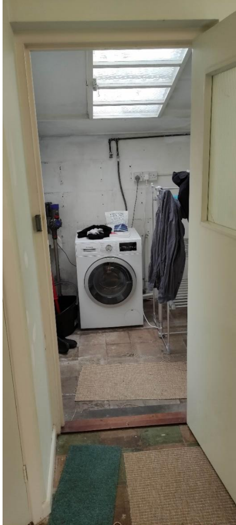
Fig.8 Internal view of the existing extension.
