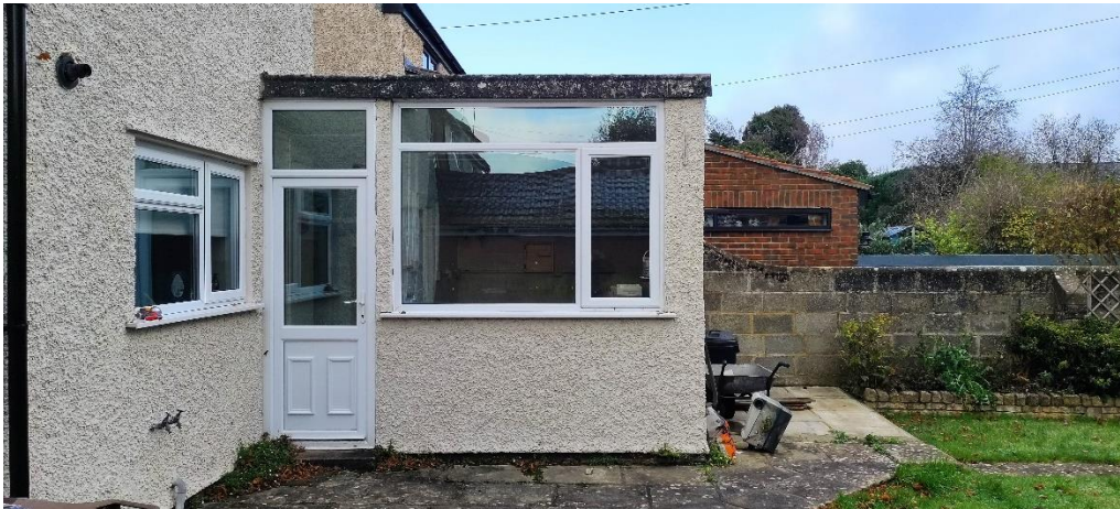
Fig.4 Closer view of the existing extension from the side.
