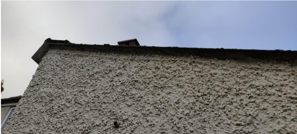
Fig.5 Detail view of the existing extension's roof edge (Rear).
