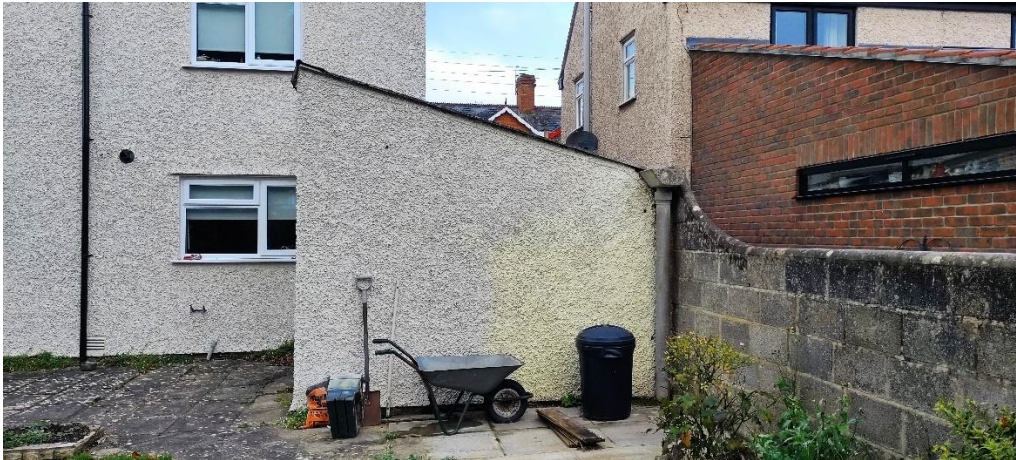
Fig.3 Closer view of the existing extension from the rear garden.
