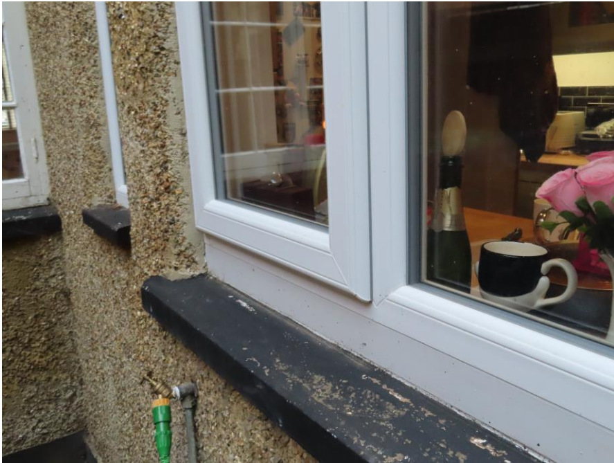
Existing Kitchen Window
