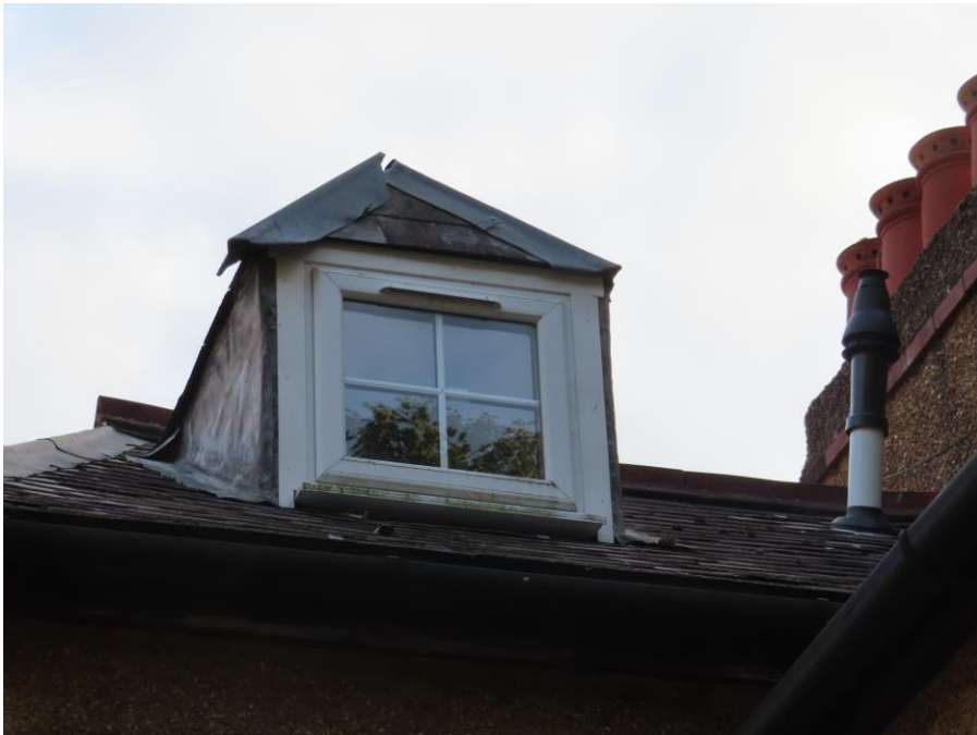
Rear Second Floor
