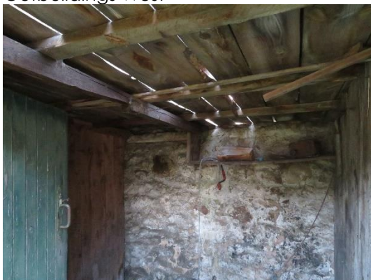
Small shed interior
