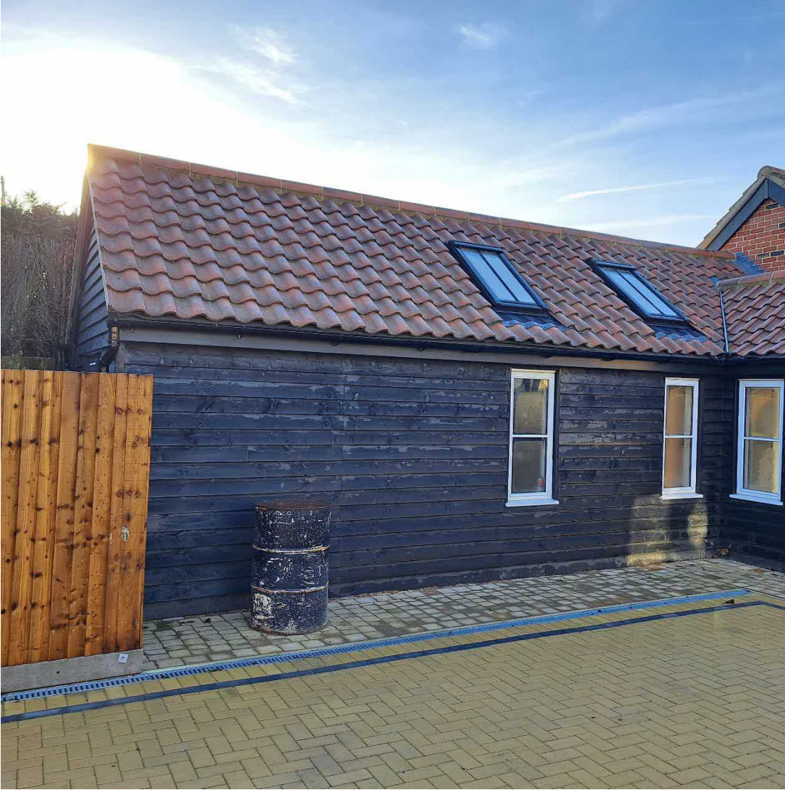
PHOTO 9 REAR VIEW NOVEMBER 2023
