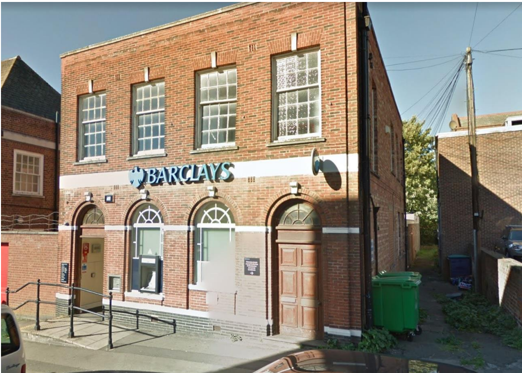
Figure 5. Street view of property. (2021).
