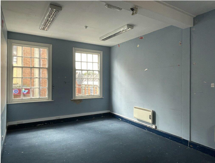
Figure 4 – photo showing large windows giving ample daylight that would be within flat 5.
