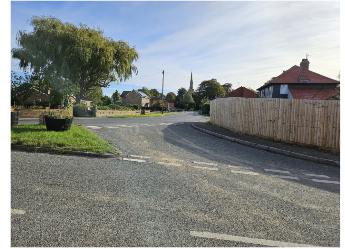
SITE PHOTOGRAPH ONE: STANDING IN RINGERS LANE LOOKING TOWARDS GOREFIELD ROAD INDICATING THE SITE BOUNDARY FENCE
