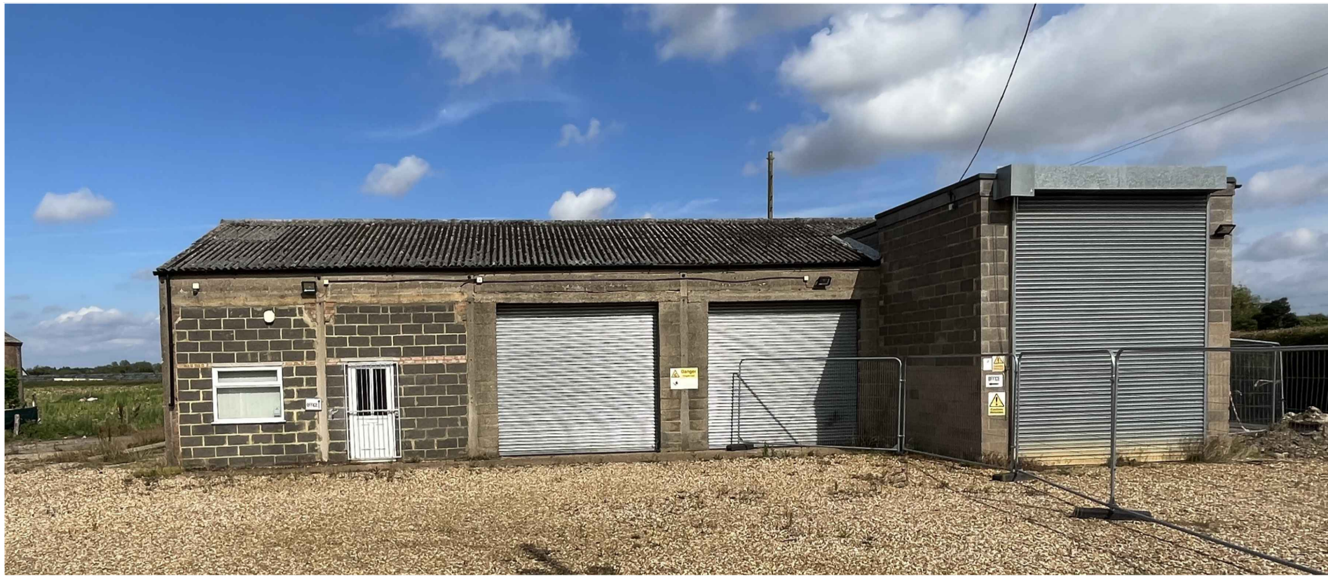
IMAGE OF FRONT ELEVATION OF EXISTING DEPOT BUILDING NTS
