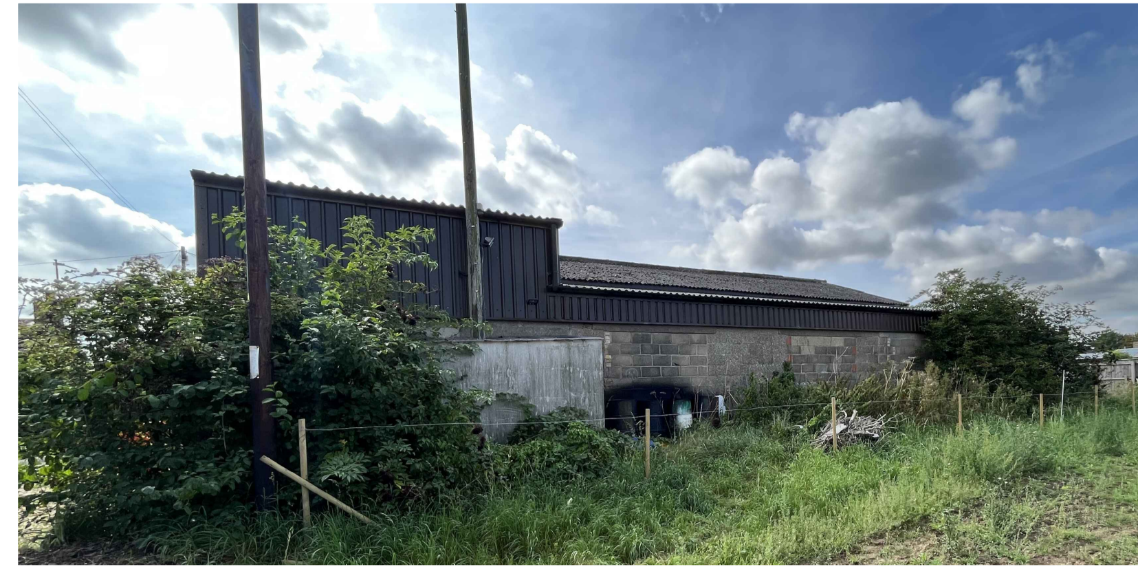
IMAGE OF REAR ELEVATION OF EXISTING DEPOT BUILDING NTS
