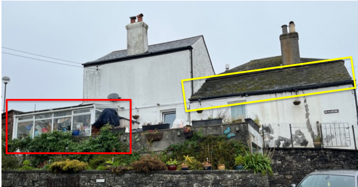
Figure 1 – Ivydene – South Elevation Conservatory - red box, roof to be impacted by the proposed works – yellow box
