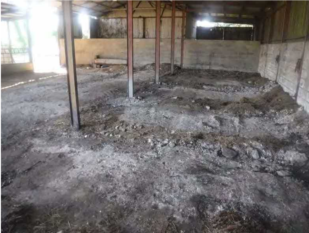
Photograph 15: Inside the on-site barn (3).
