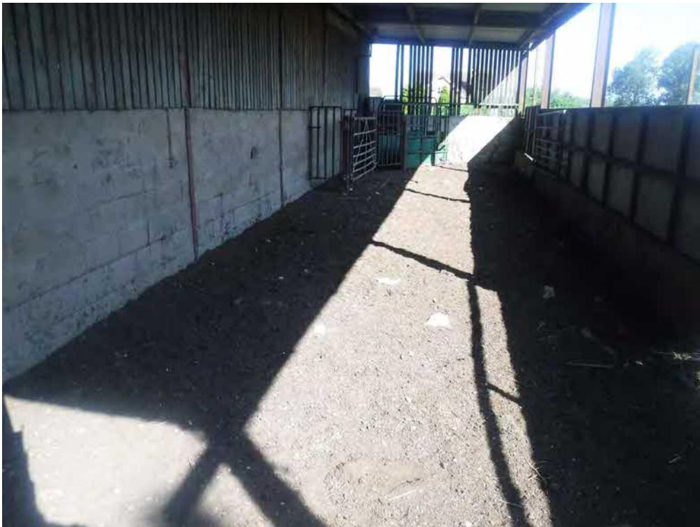
Photograph 16: Inside the on-site barn (4).
