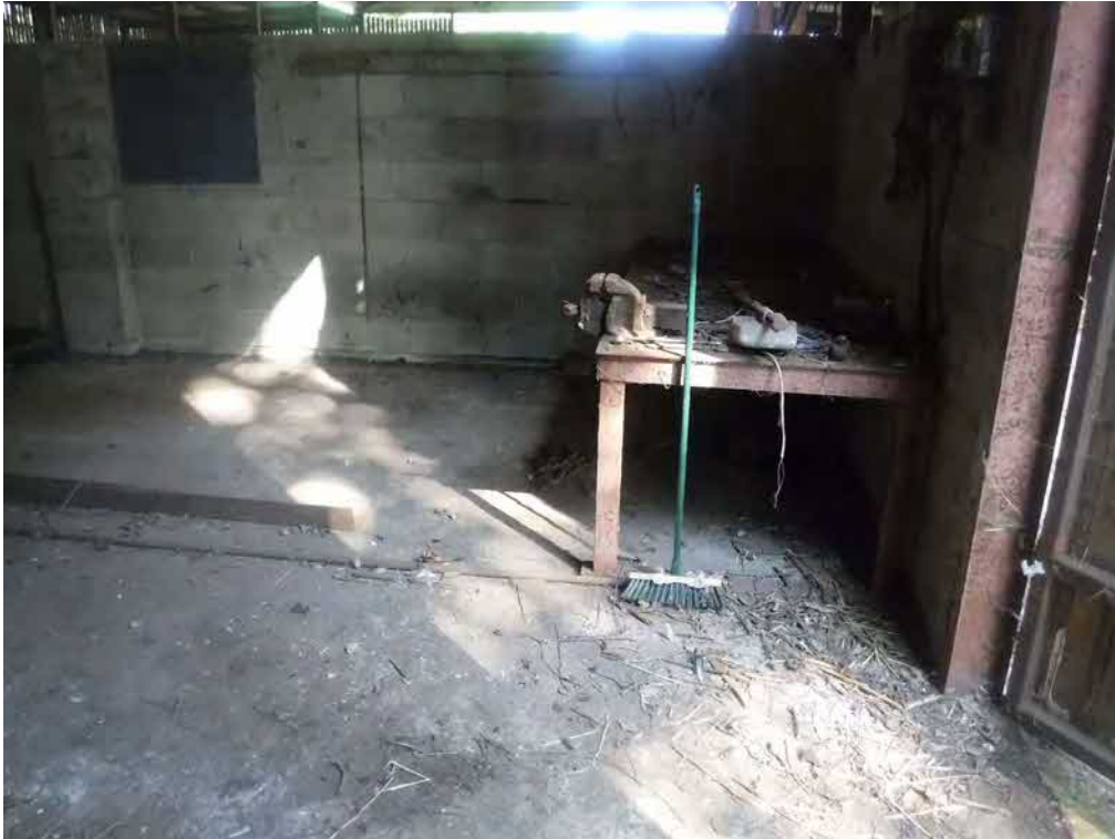
Photograph 11: Inside the workshop at the southwest end of the site (2).
