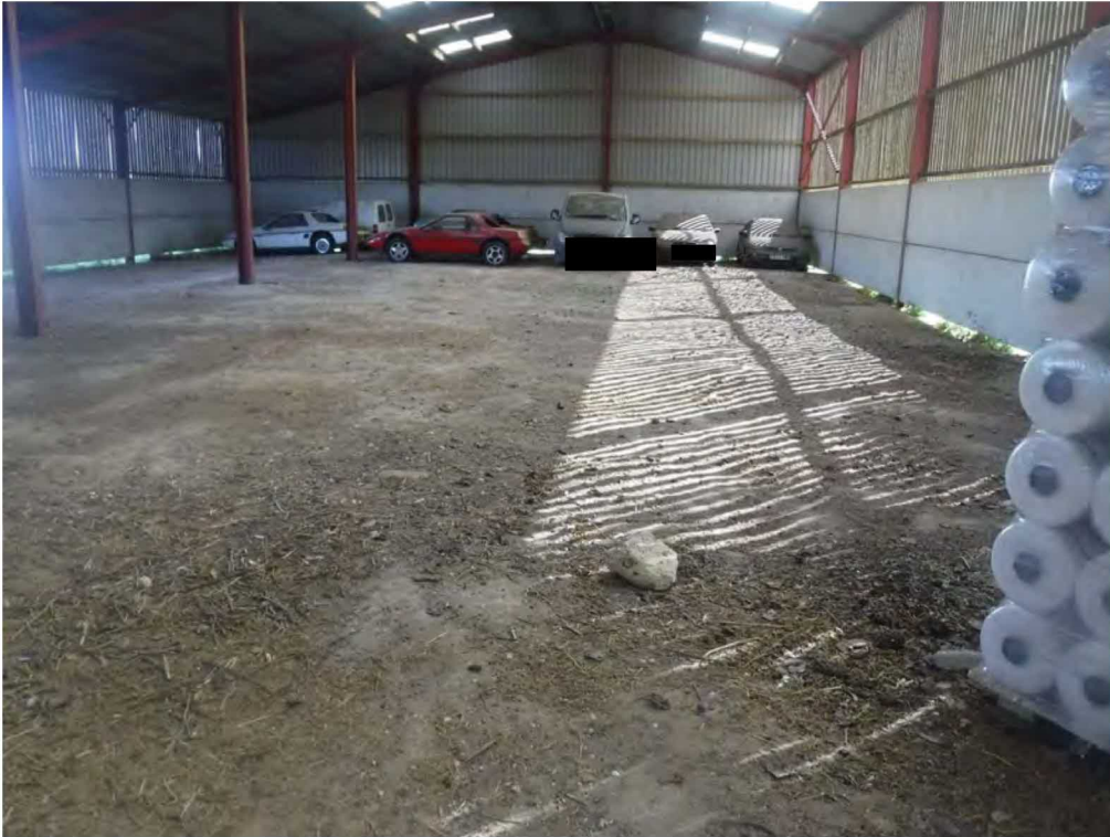
Photograph 21: Inside the modern barn (1).
