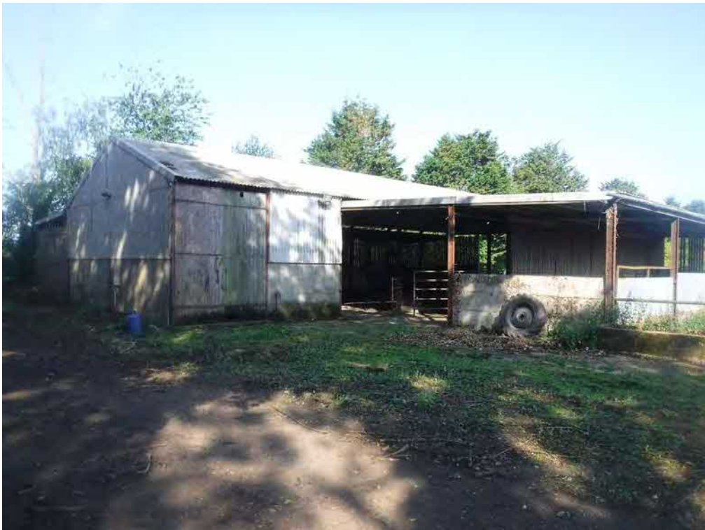
Photograph 8: The site, looking west.
