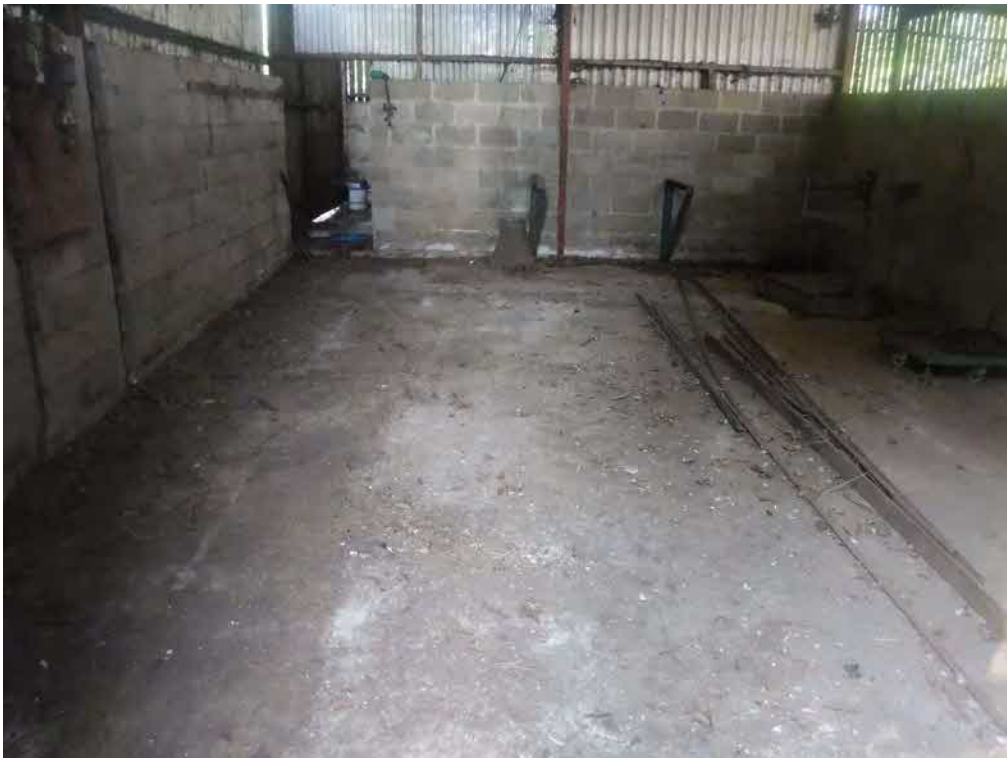
Photograph 10: Inside the workshop at the southwest end of the site (1).
