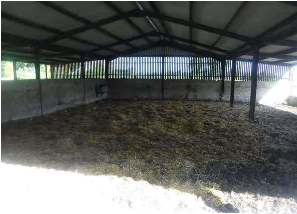
Photograph 17: Inside the off-site barn immediately to the northeast of the site.
