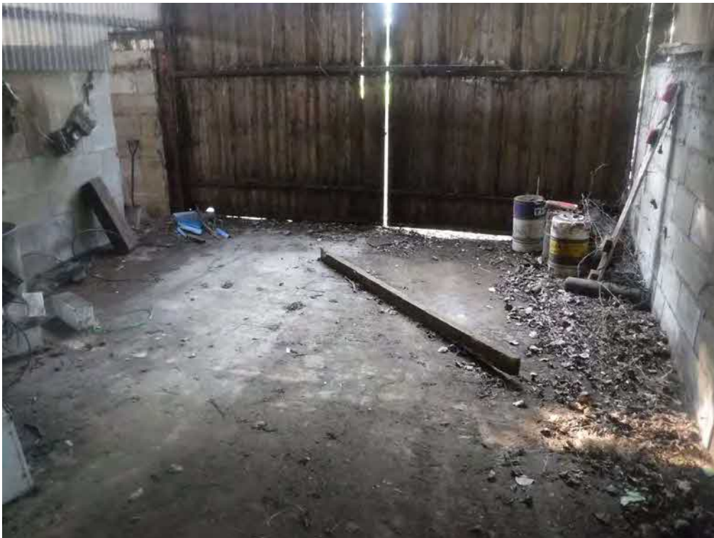
Photograph 12: Inside the workshop at the southwest end of the site (3).
