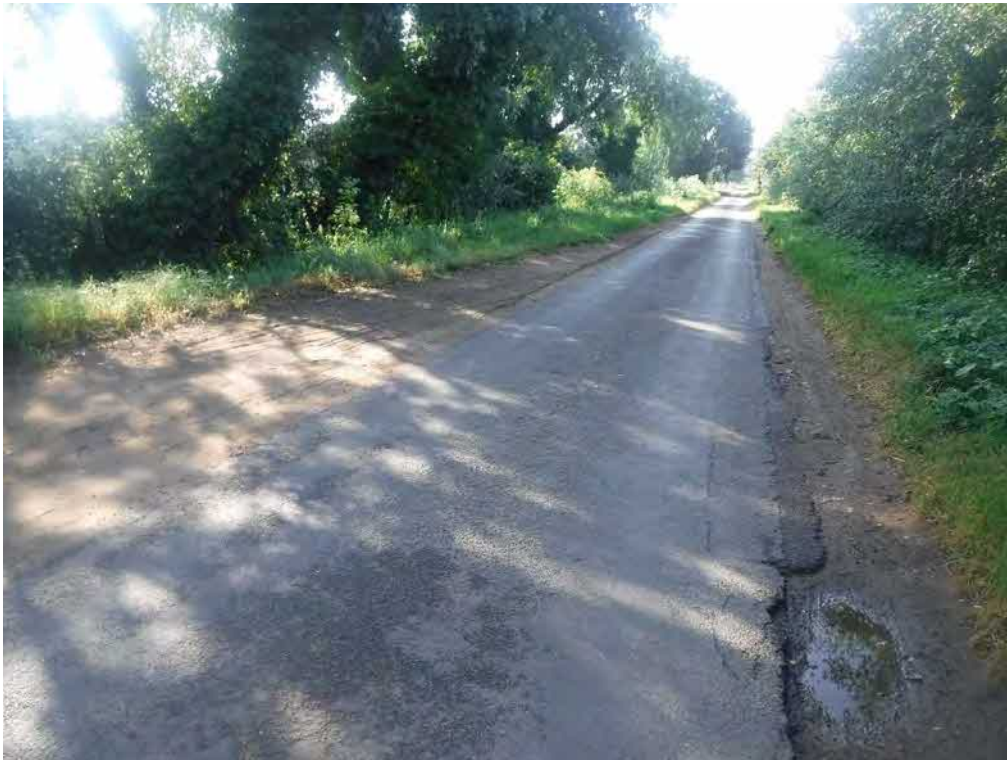
Photograph 1: Hurdle Drove looking southeast.
