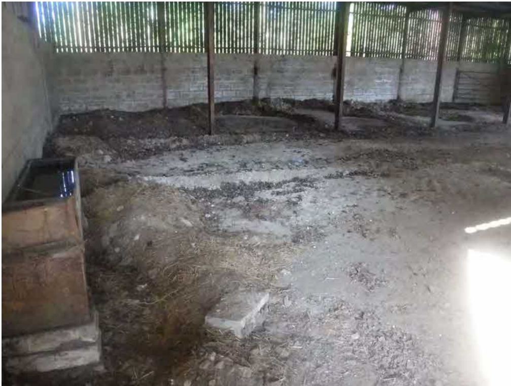
Photograph 13: Inside the on-site barn (1).
