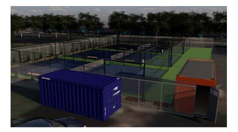
4.3 The padel court enclosure is max 4m high at the back end of the court. The court and surrounding consist of wired mesh and see-through 12mm tempered glass. There are 18 glass panels per court all 3x2 meters at the back of the court.
