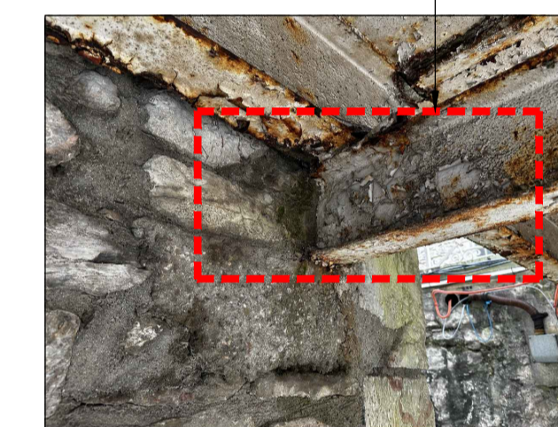
STEEL CANTILEVER BEAM FIXED INTO WALL
