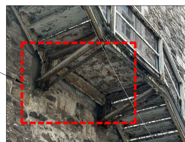
CONNECTION BETWEEN STEEL STAIRWAY AND HISTORIC WALL
