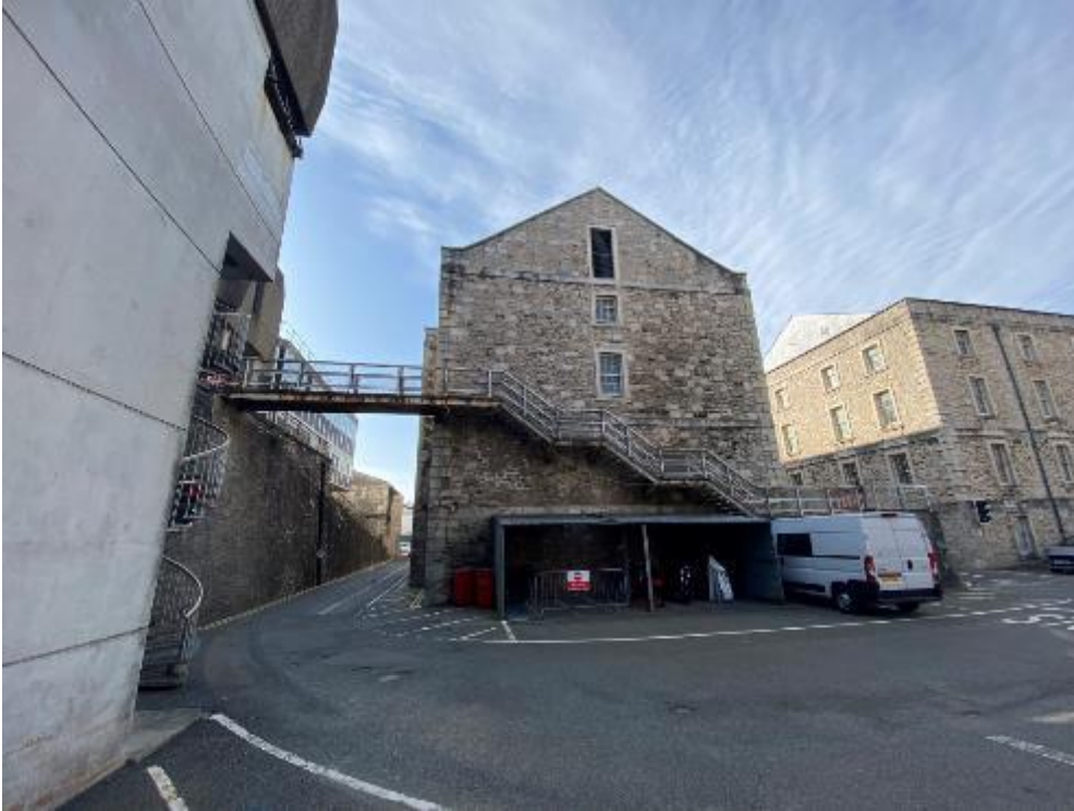
Photo 2 – View of the existing stairs supported on the external façade of the Grade II* listed building
