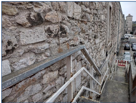
Metal gantry (looking west)
