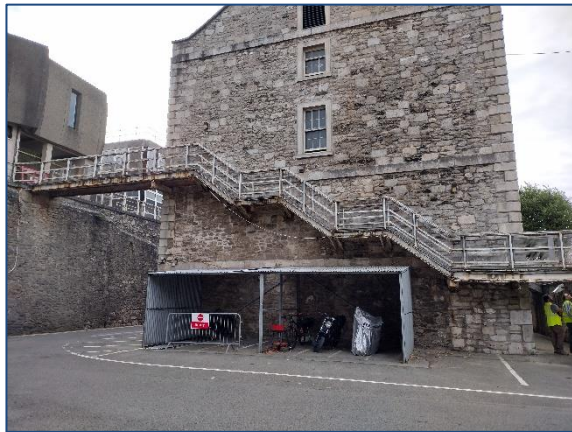
Metal gantry (north elevation)
