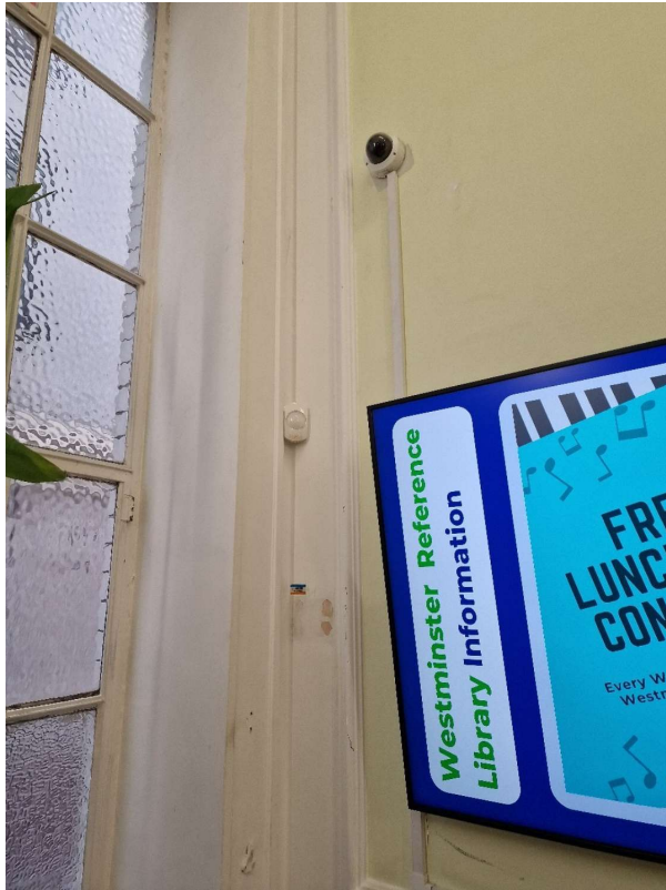
GF - Existing - Old Camera To NE Lobby Corner - To be Removed (Not on Plans)
