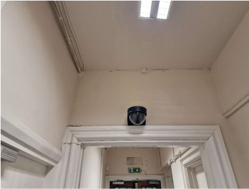
2F - Existing - CCTV To Library Work Area North Exit - To be Removed (Not on Plans)
