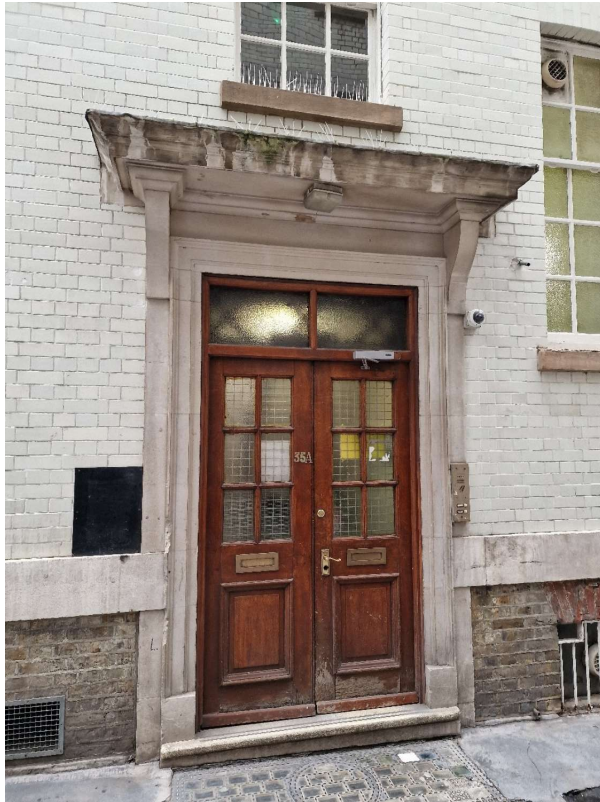
External Side Entrance - Overview
