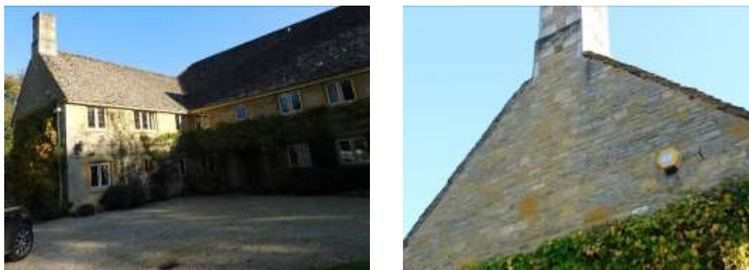
Figs. 3 & 4 Roof and northwest facing gable end
