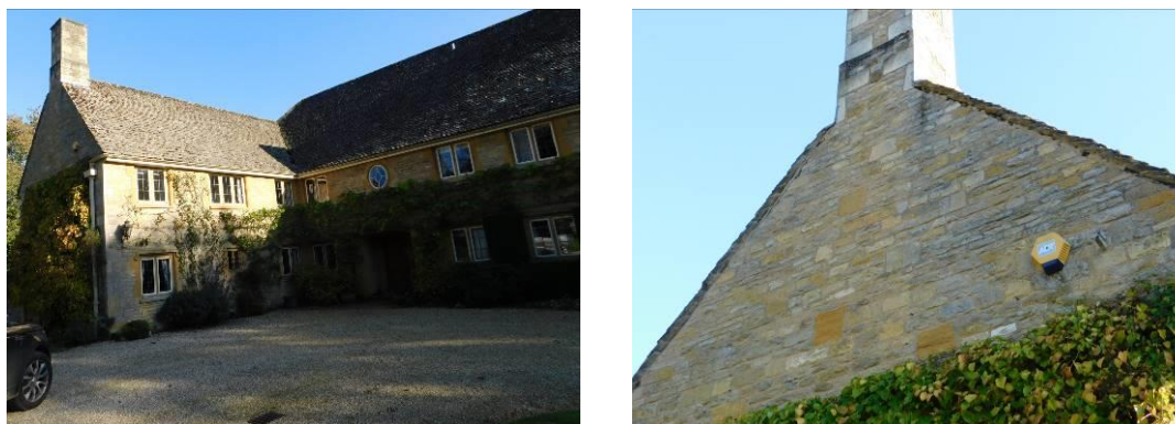
Figs. 3 & 4 Roof and northwest facing gable end
