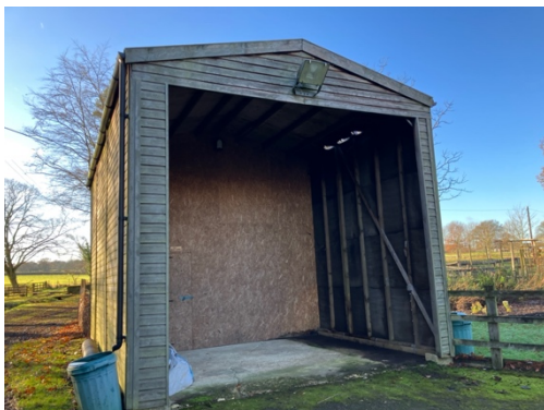
Photograph 11: Bat Mitigation Barn (B2) Open-fronted east elevation
