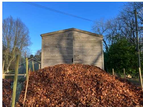
Photograph 12: Building B2, west elevation with slot access for bats
