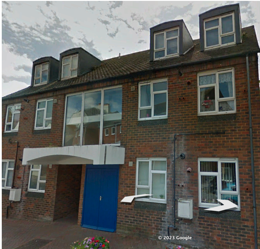
FIG 1 – No.9 New Street (grey dormers and blue, timber door)
