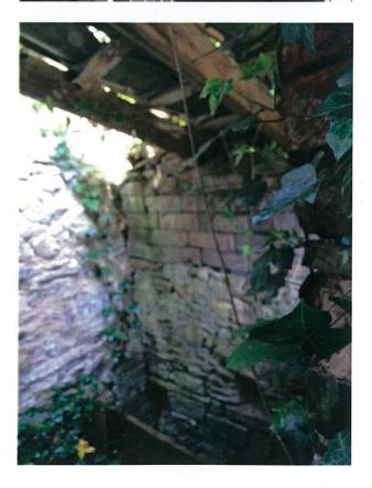
2.10 The southern lean to has a roof covered in triple roman clay tiles, and has solid masonry walls of lias.
