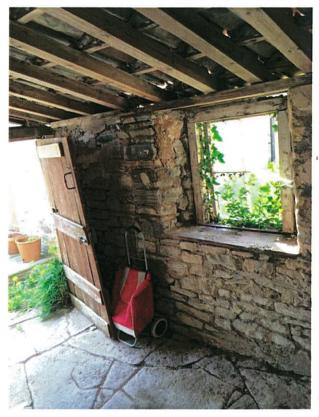
2.12 The walls to this lean to are generally plumb and stable. There is a crack in the south wall of the central building which is more visible inside the lean to. This crack should be held together by stainless steel bars glued into the bed joint either side of the movement crack.
