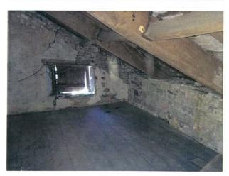
2.7 At the eaves, the rafters are bearing on a small wall plate at the outer edge of the wall. The principal rafters simply bear on top of the masonry.
