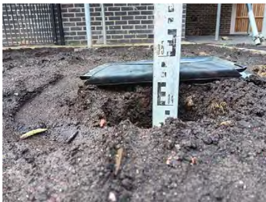
Photograph 86: View of depth of soil within the front garden of Plot 48.
