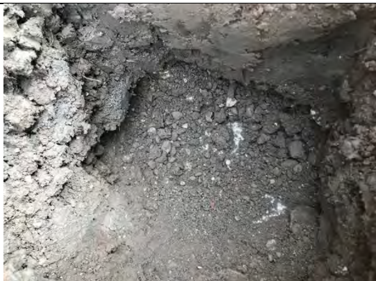
Photograph 142: View of soil within cover system and geotextile at base in front of Plots 58/59.
