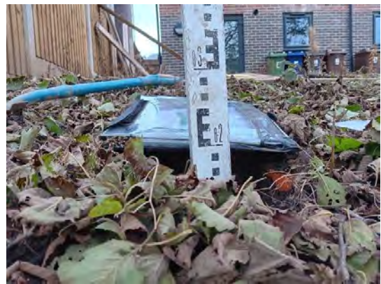
Photograph 17: View of depth of soil within the rear (S) garden of Plot 38.
