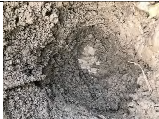
Photograph 163: View of soil within cover system and geotextile at base in front of Plot 62.
