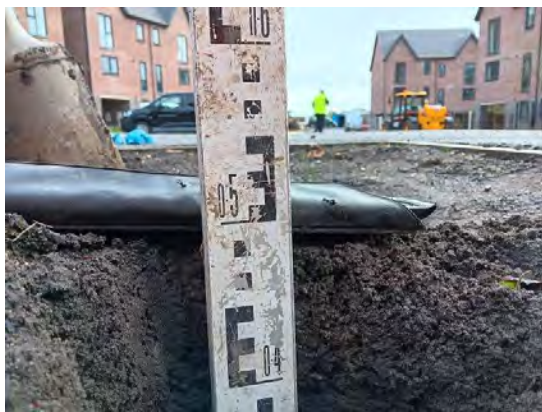
Photograph 74: View of depth of soil within the front garden of Plot 46.
