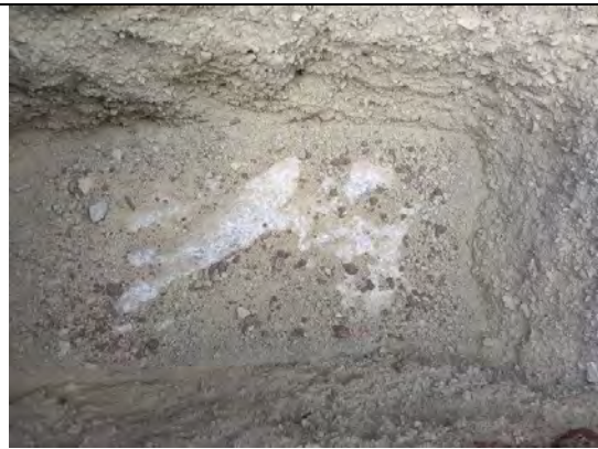
Photograph 66: View of soil within cover system and geotextile at base in rear of Plot 44.
