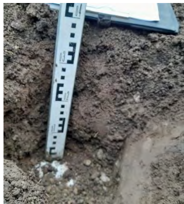
Photograph 62: View of depth of soil within the front garden of Plot 44.
