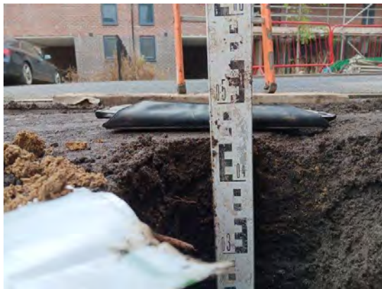
Photograph 68: View of depth of soil within the front garden of Plot 45.
