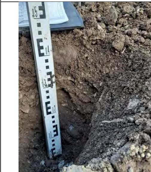
Photograph 20: View of depth of soil within the front garden of Plot 39.
