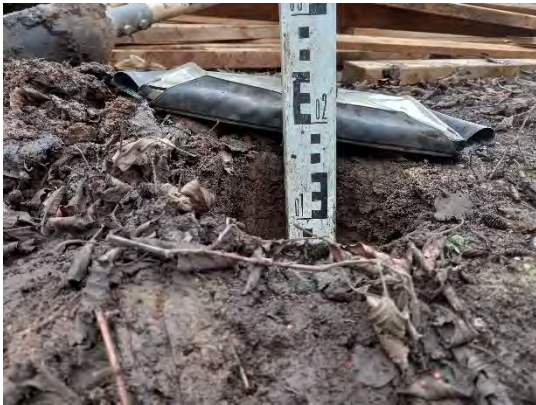
Photograph 188: View of depth of soil within the shared soft landscaping B4.
