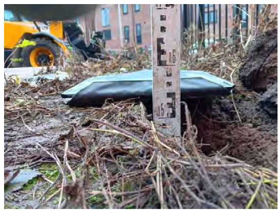
Photograph 11: View of depth of soil within the front garden of Plot 38.
