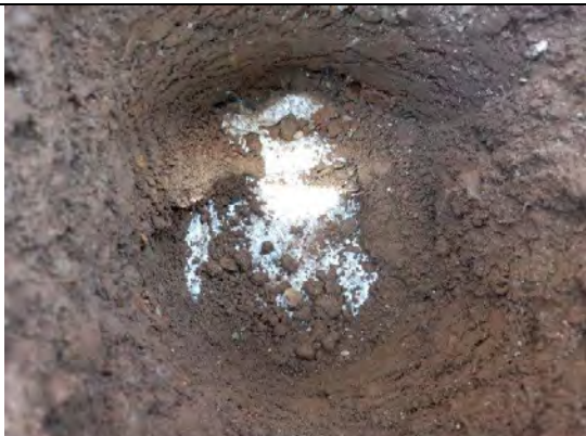
Photograph 45: View of soil within cover system and geotextile at base in rear (S) of Plot 41.
