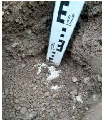
Photograph 63: View of soil within cover system and geotextile at base in front of Plot 44.
