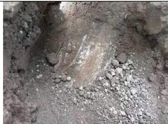
Photograph 42: View of soil within cover system and geotextile at base in rear (N) of Plot 41.
