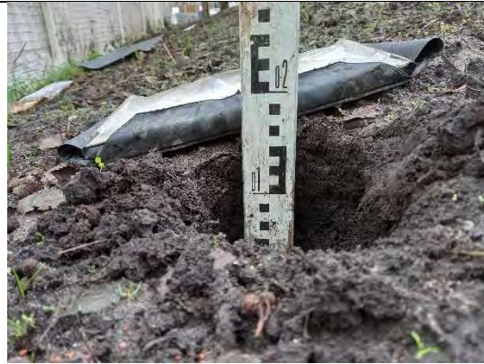
Photograph 185: View of depth of soil within the shared soft landscaping B3.
