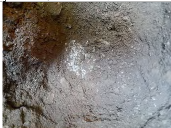
Photograph 3: View of soil within cover system and geotextile at base in front of Plot 37.
