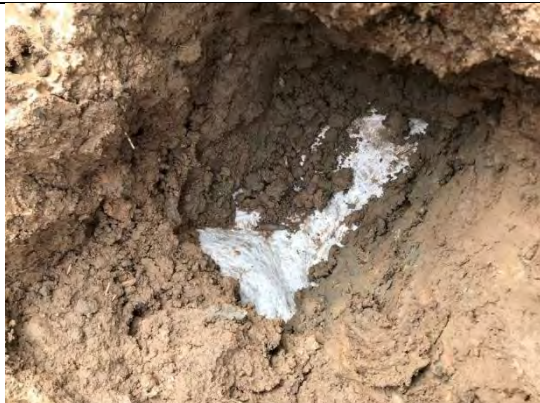
Photograph 136: View of soil within cover system and geotextile at base in front of Plots 57/58.
