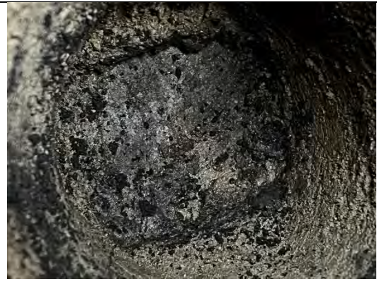
Photograph 102: View of soil within cover system and geotextile at base in rear of Plot 50.
