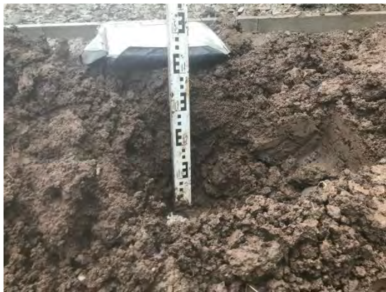
Photograph 119: View of depth of soil within the front gardens of Plot 54/55.
