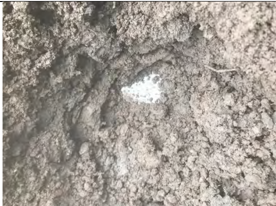
Photograph 120: View of soil within cover system and geotextile at base in front of Plots 54/55.
