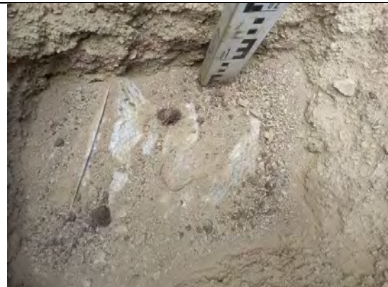
Photograph 60: View of soil within cover system and geotextile at base in rear of Plot 43.
