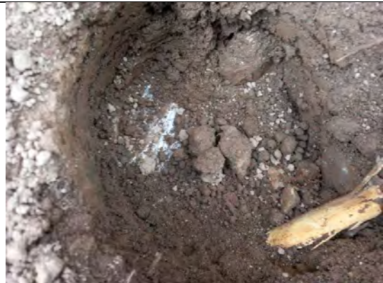
Photograph 54: View of soil within cover system and geotextile at base in rear (S) of Plot 42.
