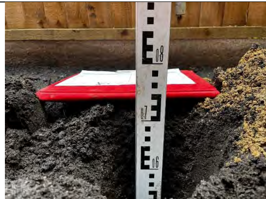
Photograph 108: View of soil within cover system and geotextile at base in rear of Plot 51.
