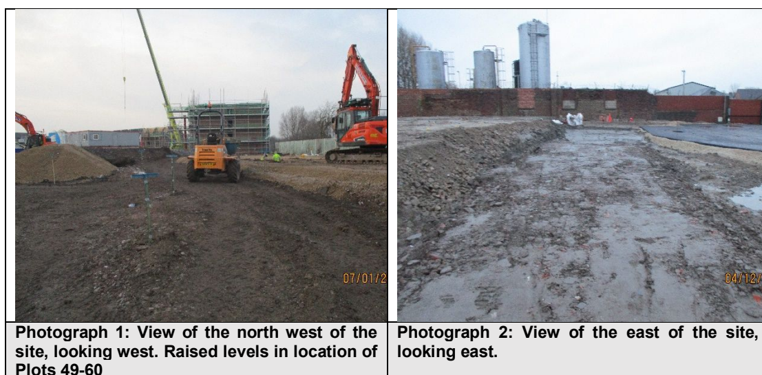
Plate 1-2: Site photographs taken during earthworks.
