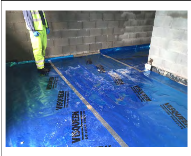
Photograph 1: Evidence of gas membrane coverage across Plot 57.
