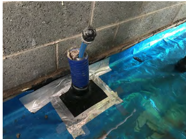
Photograph 2: Evidence of appropriate sealing around services for Plot 54.
