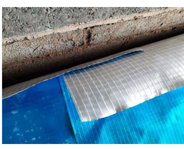
Photograph 4: Evidence of appropriate overlap of the membrane for Plot 2.
