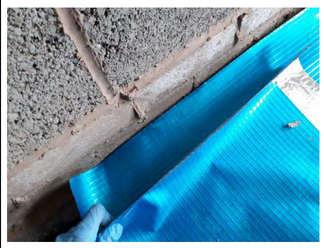
Photograph 4: Evidence of appropriate overlap of the membrane for Plot 42.
