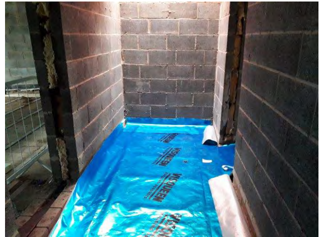
Photograph 2: Evidence of gas membrane coverage across corridor.
