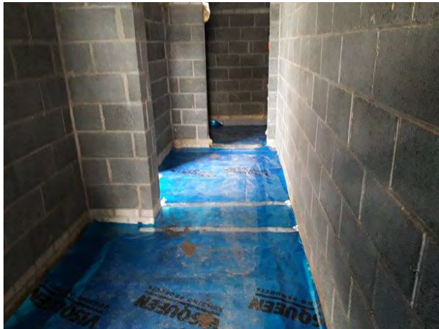
Photograph 3: Evidence of gas membrane coverage across corridor.
