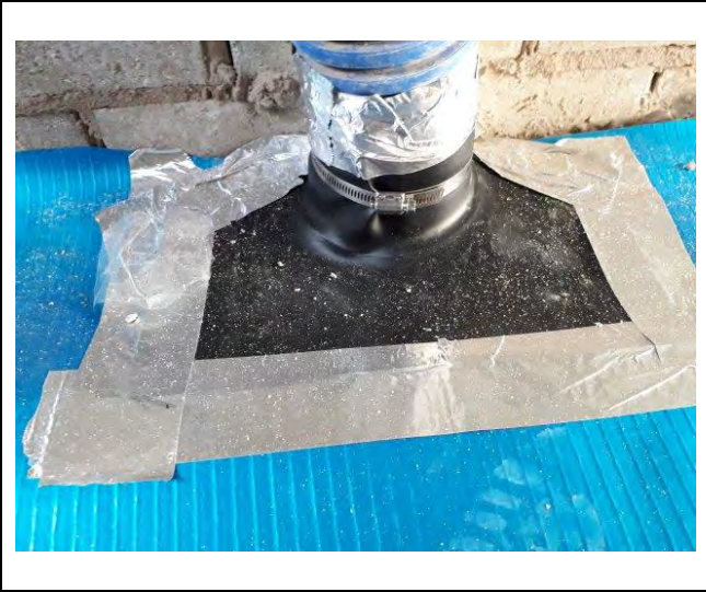
Photograph 2: Evidence of appropriate sealing around services for Plot 42.
