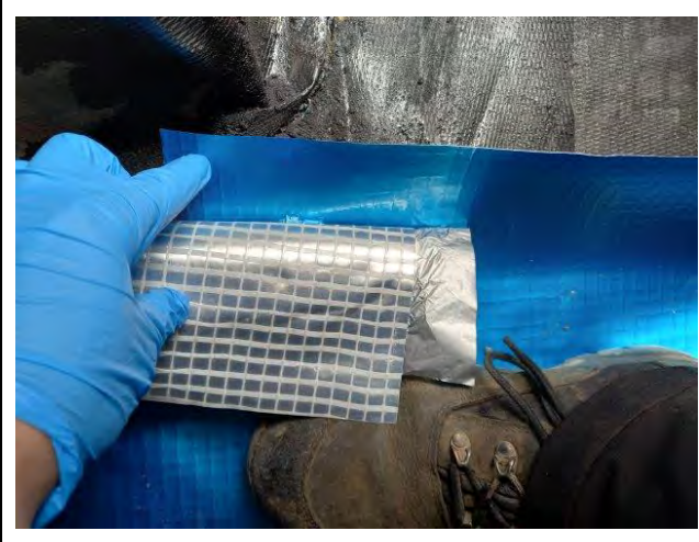
Photograph 4: Evidence of appropriate overlap of the membrane for Plot 62.
