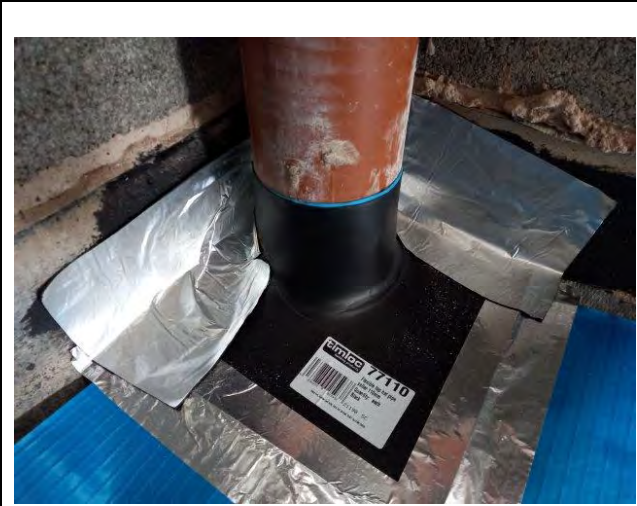
Photograph 2: Evidence of appropriate sealing around services for Plot 62.
