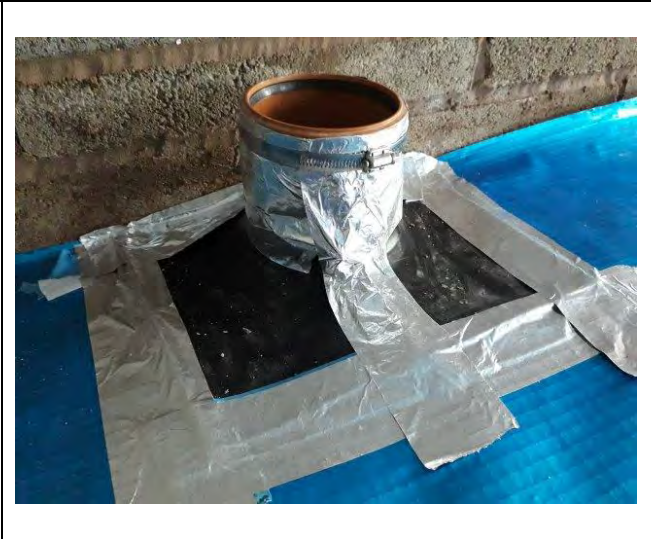
Photograph 2: Evidence of appropriate sealing around services for Plot 8.
