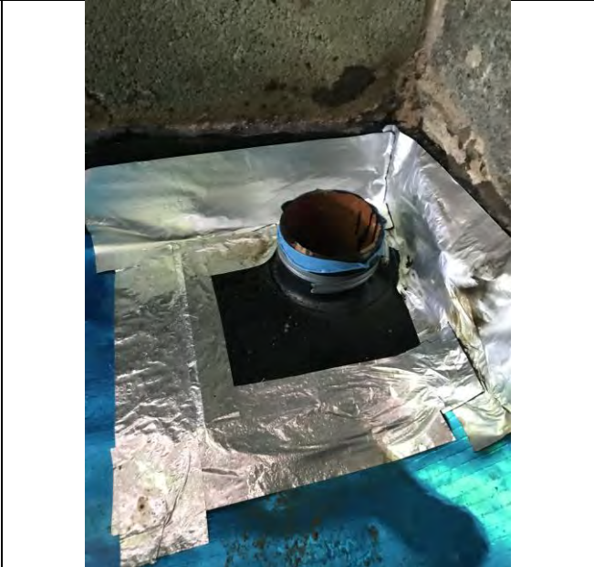
Photograph 2: Evidence of appropriate sealing around services for Plot 56.
