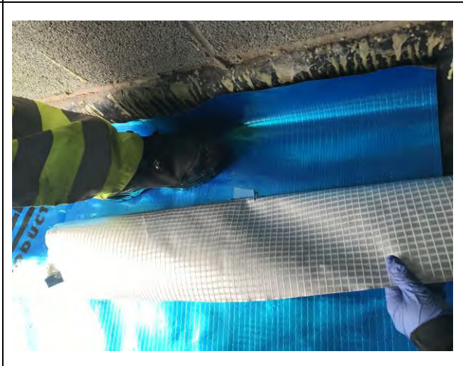
Photograph 4: Evidence of appropriate overlap of the membrane for Plot 55.
