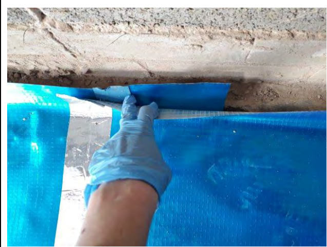
Photograph 4: Evidence of appropriate overlap of the membrane for Plot 37.
