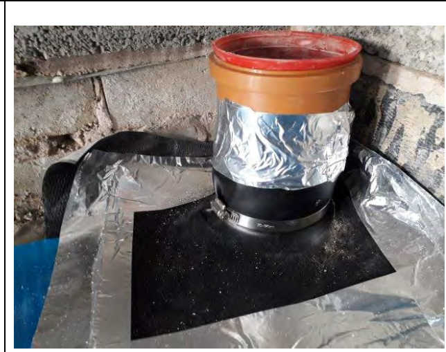
Photograph 2: Evidence of appropriate sealing around services for Plot 43.
