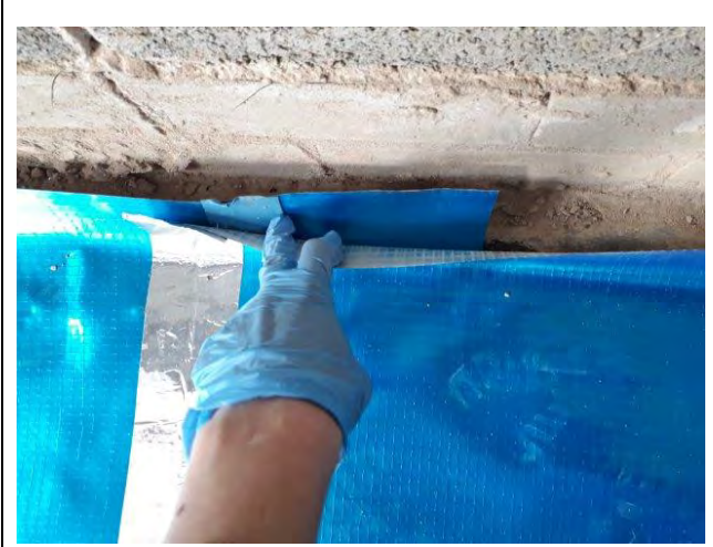
Photograph 4: Evidence of appropriate overlap of the membrane for Plot 45.
