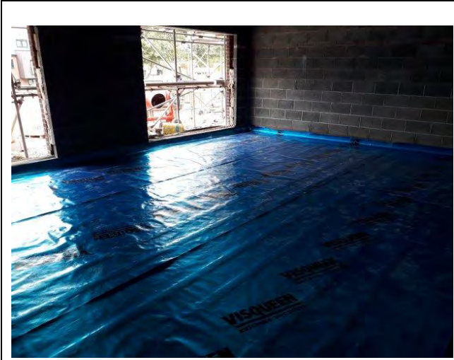
Photograph 1: Evidence of gas membrane coverage across Plot 3.
