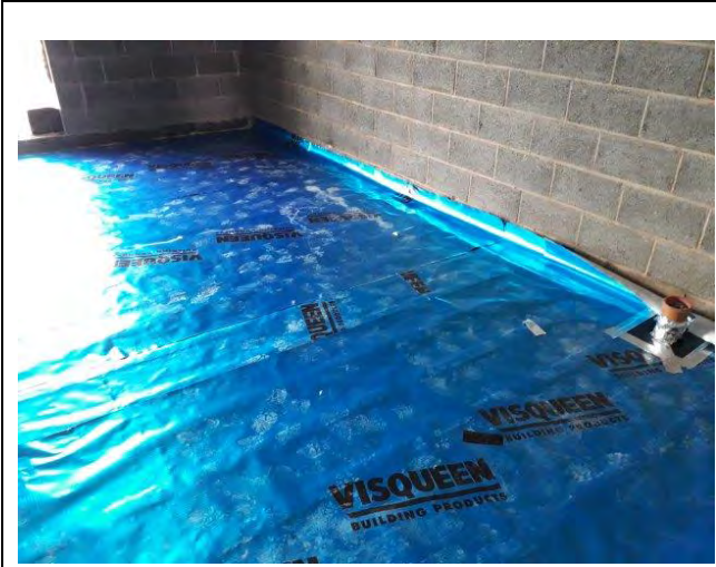
Photograph 1: Evidence of gas membrane coverage across Plot 2.
