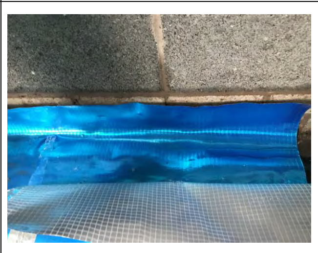
Photograph 4: Evidence of appropriate overlap of the membrane for Plot 53.
