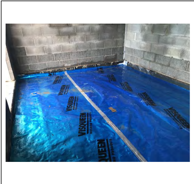
Photograph 1: Evidence of gas membrane coverage across Plot 53.
