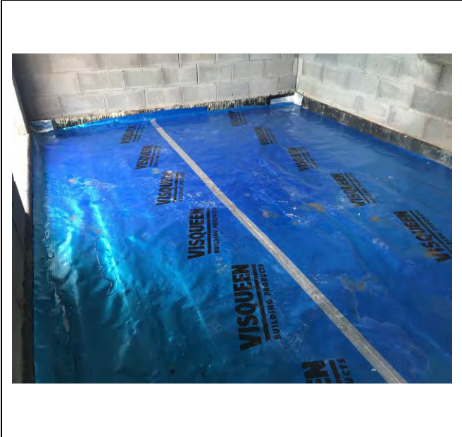
Photograph 1: Evidence of gas membrane coverage across Plot 56.
