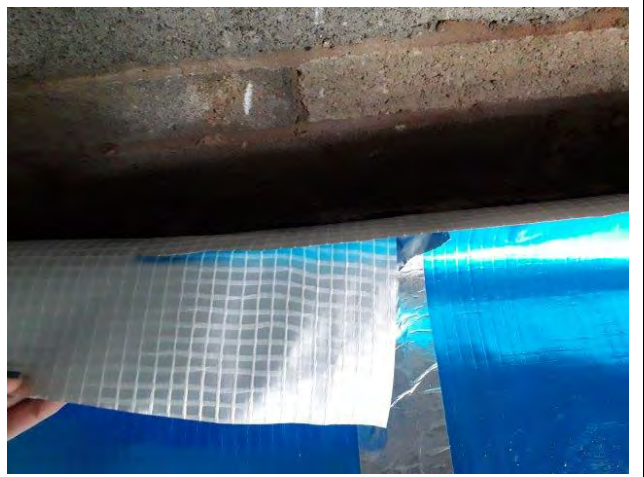
Photograph 4: Evidence of appropriate overlap of the membrane for Plot 4.
