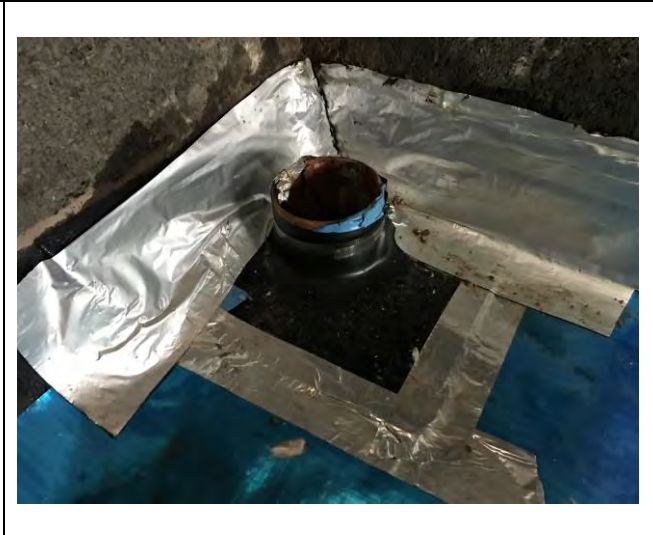
Photograph 2: Evidence of appropriate sealing around services for Plot 57.
