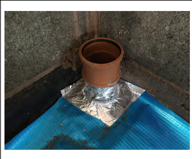
Photograph 2: Evidence of appropriate sealing around services for Plot 45.
