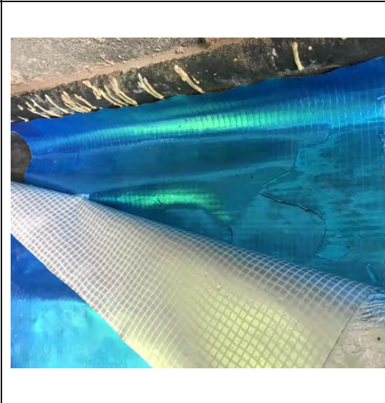
Photograph 4: Evidence of appropriate overlap of the membrane for Plot 51.
