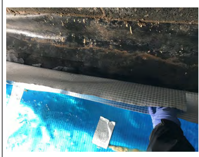
Photograph 4: Evidence of appropriate overlap of the membrane for Plot 59.
