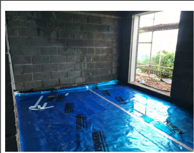
Photograph 1: Evidence of gas membrane coverage across Plot 59.
