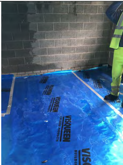
Photograph 1: Evidence of gas membrane coverage across Plot 54.
