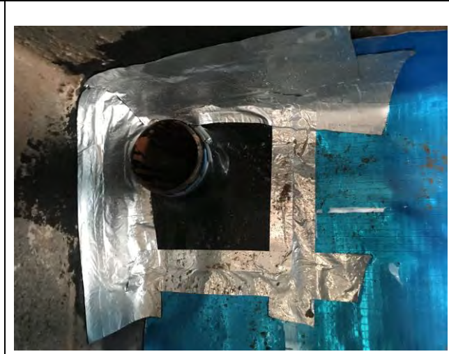
Photograph 2: Evidence of appropriate sealing around services for Plot 59.
