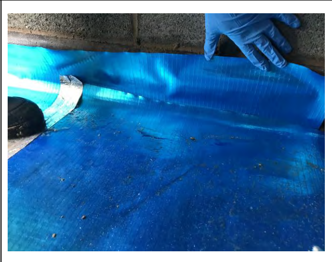
Photograph 4: Evidence of appropriate overlap of the membrane for Plot 52.
