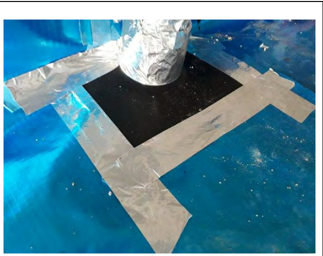
Photograph 2: Evidence of appropriate sealing around services for Plot 9.
