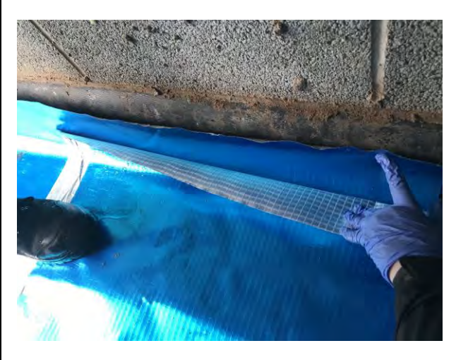
Photograph 4: Evidence of appropriate overlap of the membrane for Plot 50.
