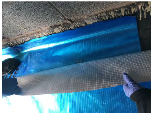
Photograph 4: Evidence of appropriate overlap of the membrane for Plot 54.
