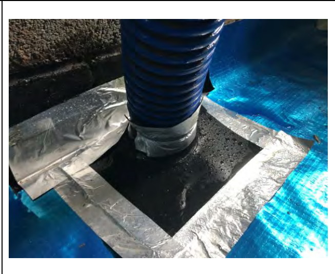
Photograph 2: Evidence of appropriate sealing around services for Plot 58.
