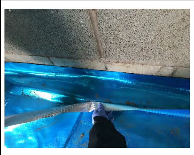
Photograph 4: Evidence of appropriate overlap of the membrane for Plot 49.
