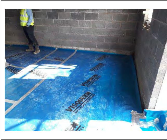
Photograph 1: Evidence of gas membrane coverage across Plot 42.
