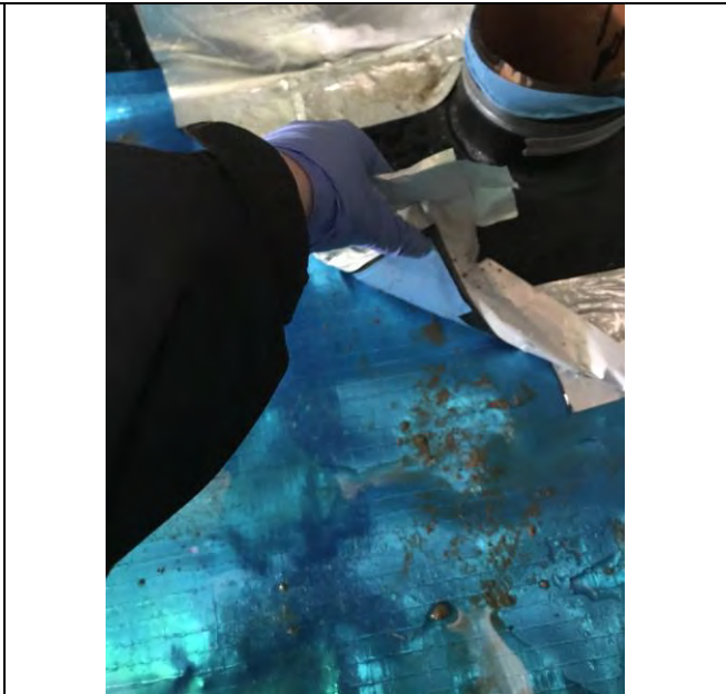
Photograph 2: Evidence of appropriate sealing around services for Plot 55.
