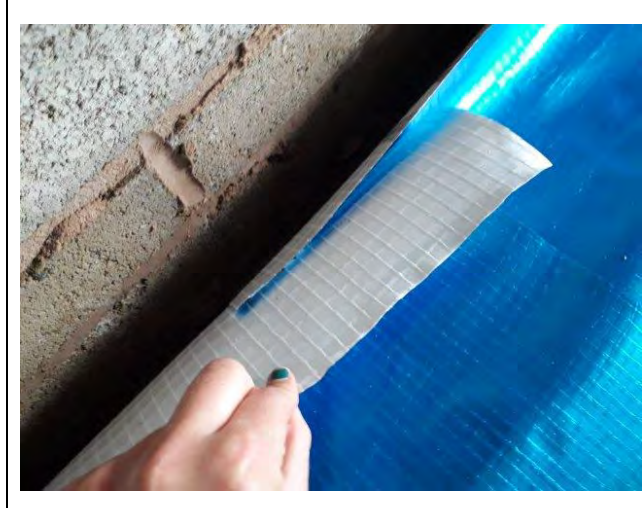
Photograph 4: Evidence of appropriate overlap of the membrane for Plot 3.
