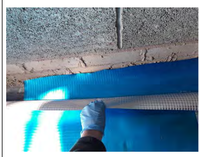
Photograph 4: Evidence of appropriate overlap of the membrane for Plot 43.
