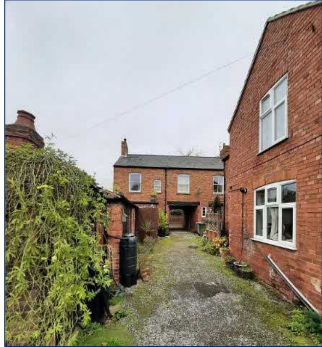
Figure 3 – View north towards no. 4 and 6 Burgage Lane
