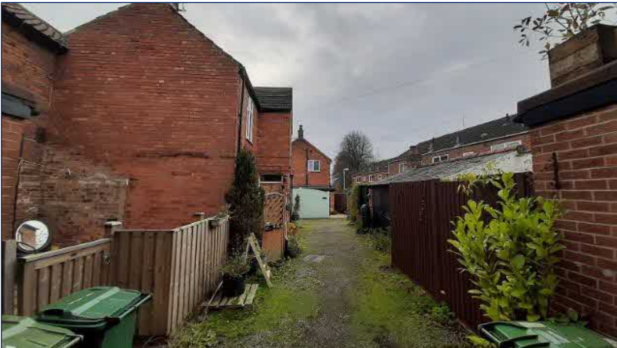
Figure 6 – View from site entrance
