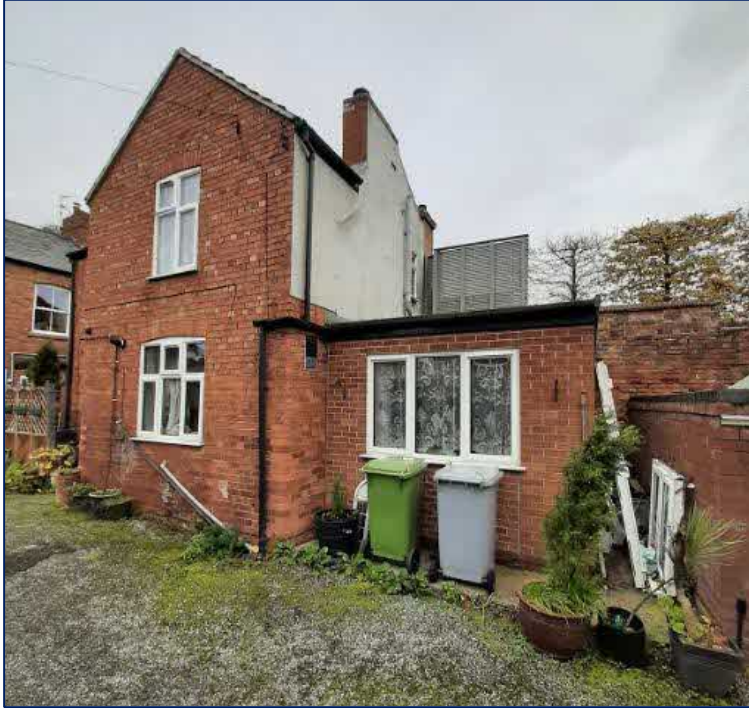
Figure 2 – Side extension at 8 Burgage Lane
