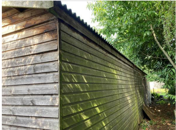
Rear of timber stable B2
