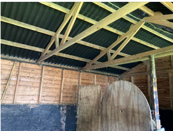
Interior of timber stable B2
