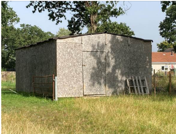
Timber framed and clad store B5
