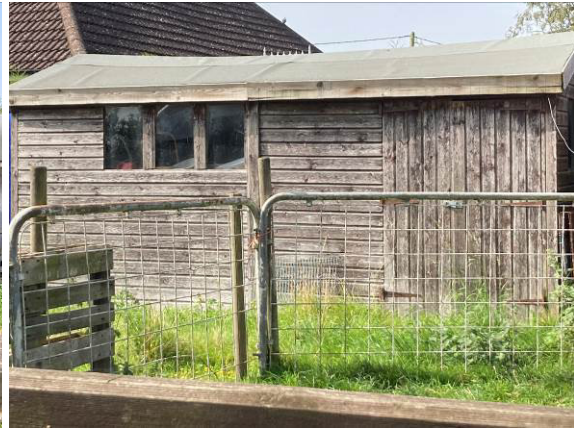
Timber framed outbuilding B4
