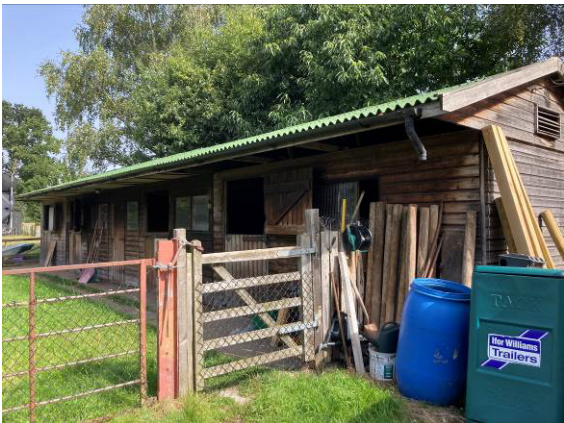
Timber stable B2
