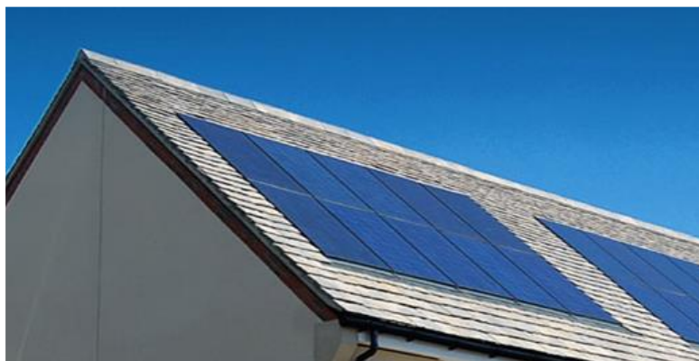
Figure 9: Typical PV installation to pitched roof
