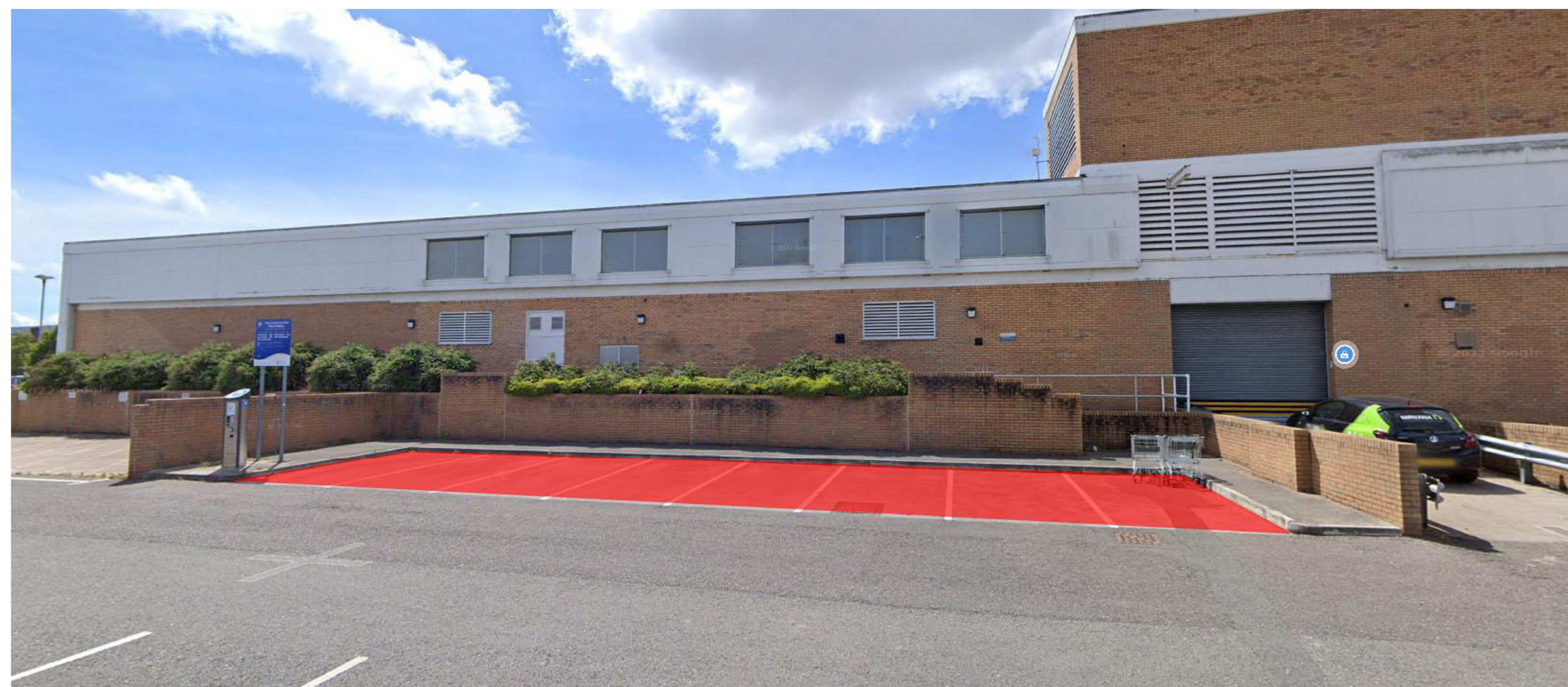
Existing parking identified for use
