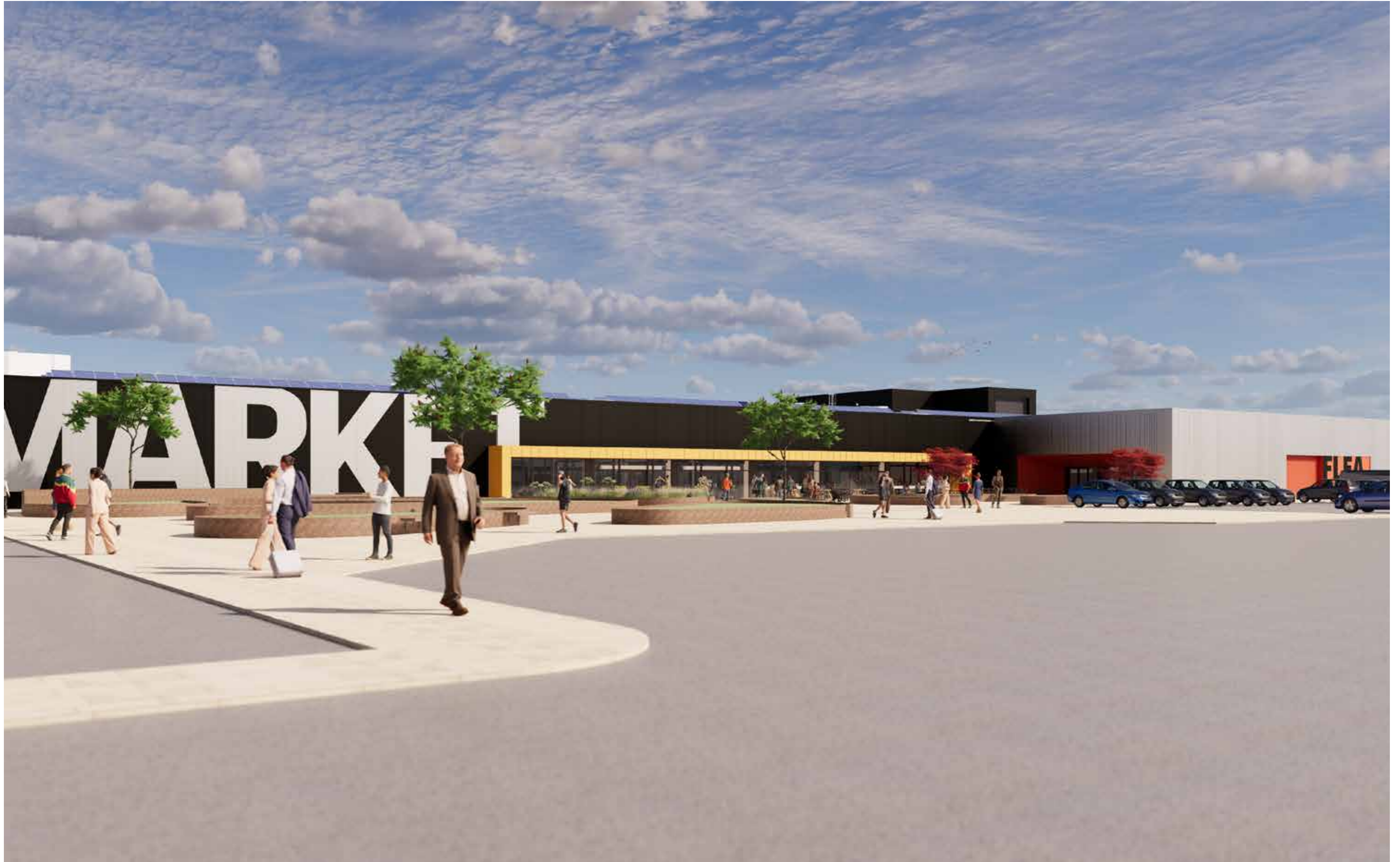
Artists Impression of the remodelling market (please note the landscape scheme is indicative and will not form part of the planning application)
