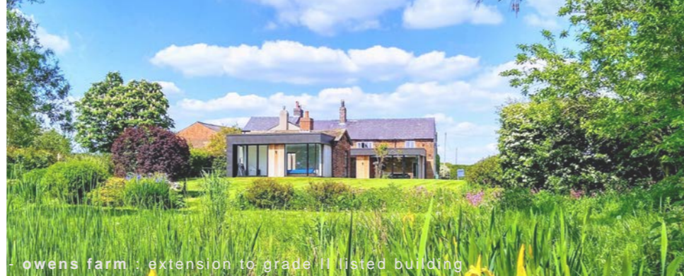
- marlewood : extension in a conservation area [West Lancs Design Awards Shortlist 2019]
