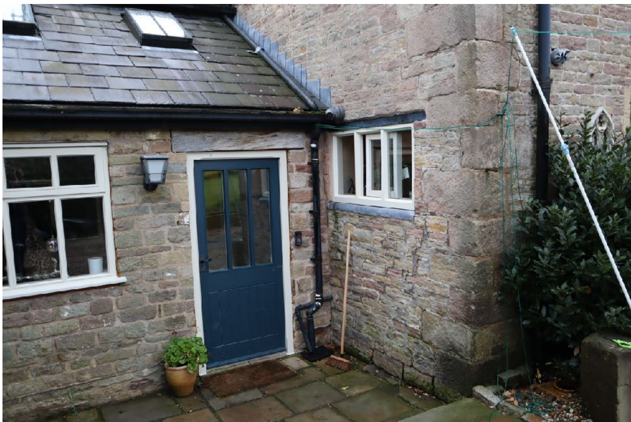
Plate 1: Modern rear extension to which the glass link will provide access. The wind pictures right will be opened up and returned to a doorway.
