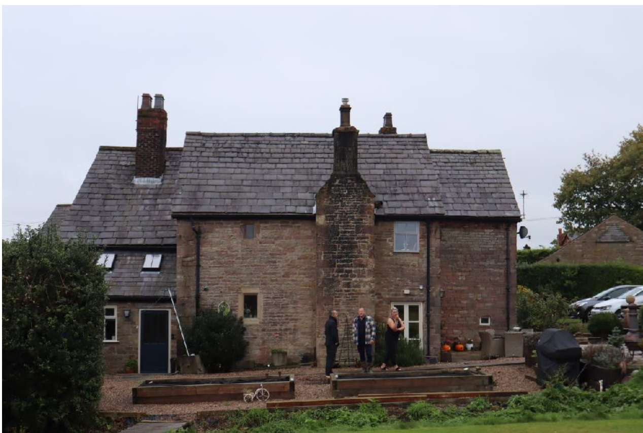
Plate 2: Western elevation where the proposed extension is to be sited.
