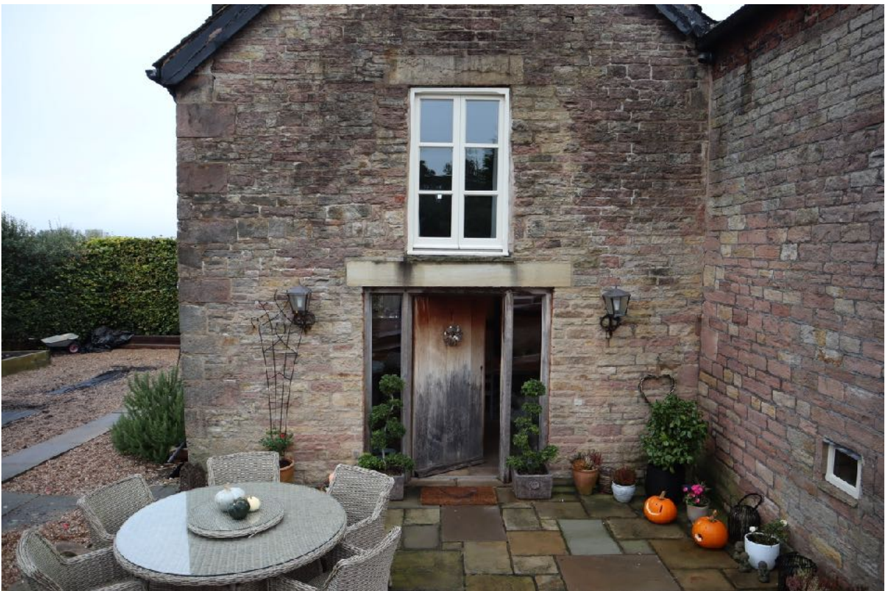
Plate 4: Site of the former granary steps and offset door to parlour access.
