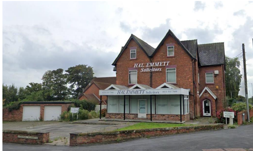
Figure 2 – Street view of the property from Liverpool Road North.
