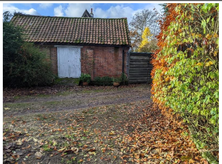
Photo 6 Garage where the battery storage unit will be located
