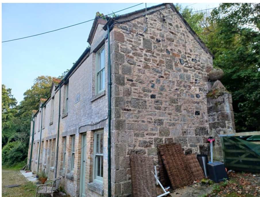
Figure 4: North and east elevations of cottages at Trereife House.
