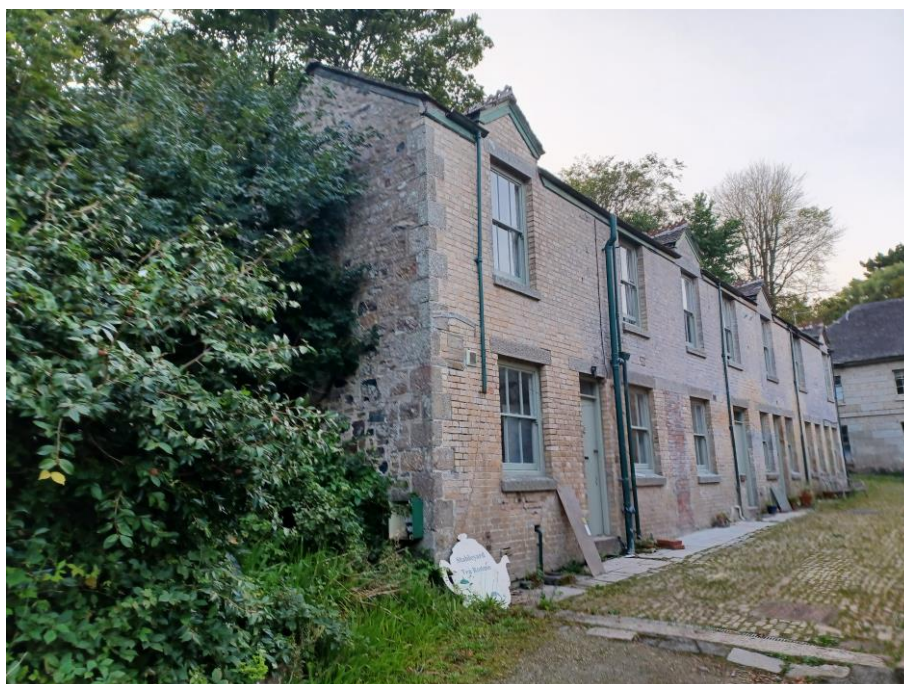
Figure 3: East and south elevations of cottages at Trereife House.
