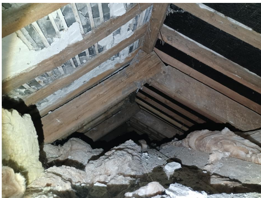
Figure 6: View of roof void within cottages at Trereife House.
