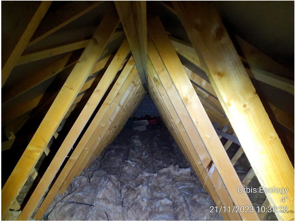
Interior of roof void
