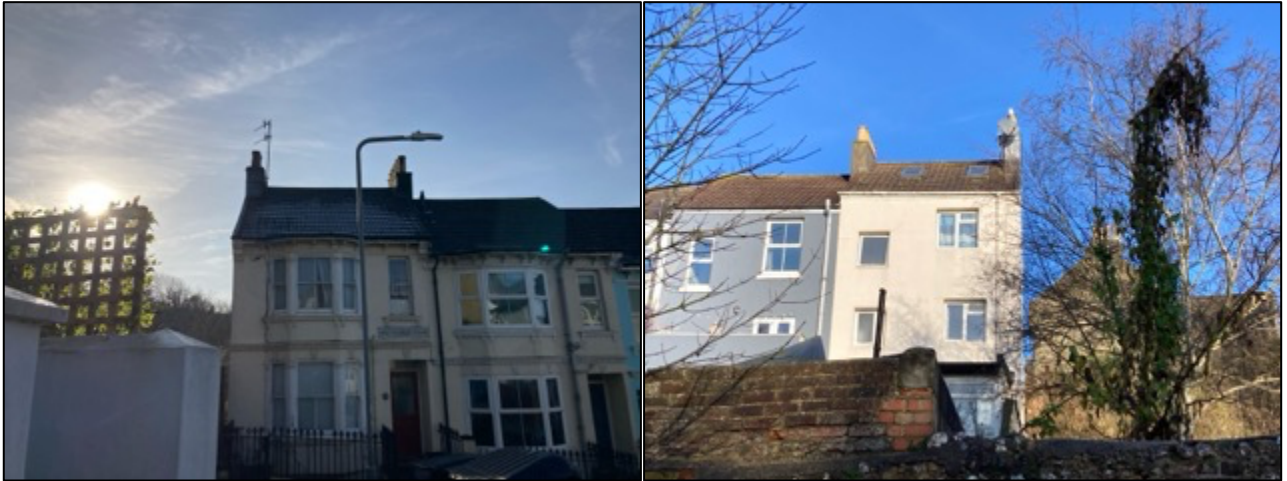
Photographs 1a (left) and 1b (right). 1a: the front (northern) aspect of the building. 1b: the rear (southern) aspect.
