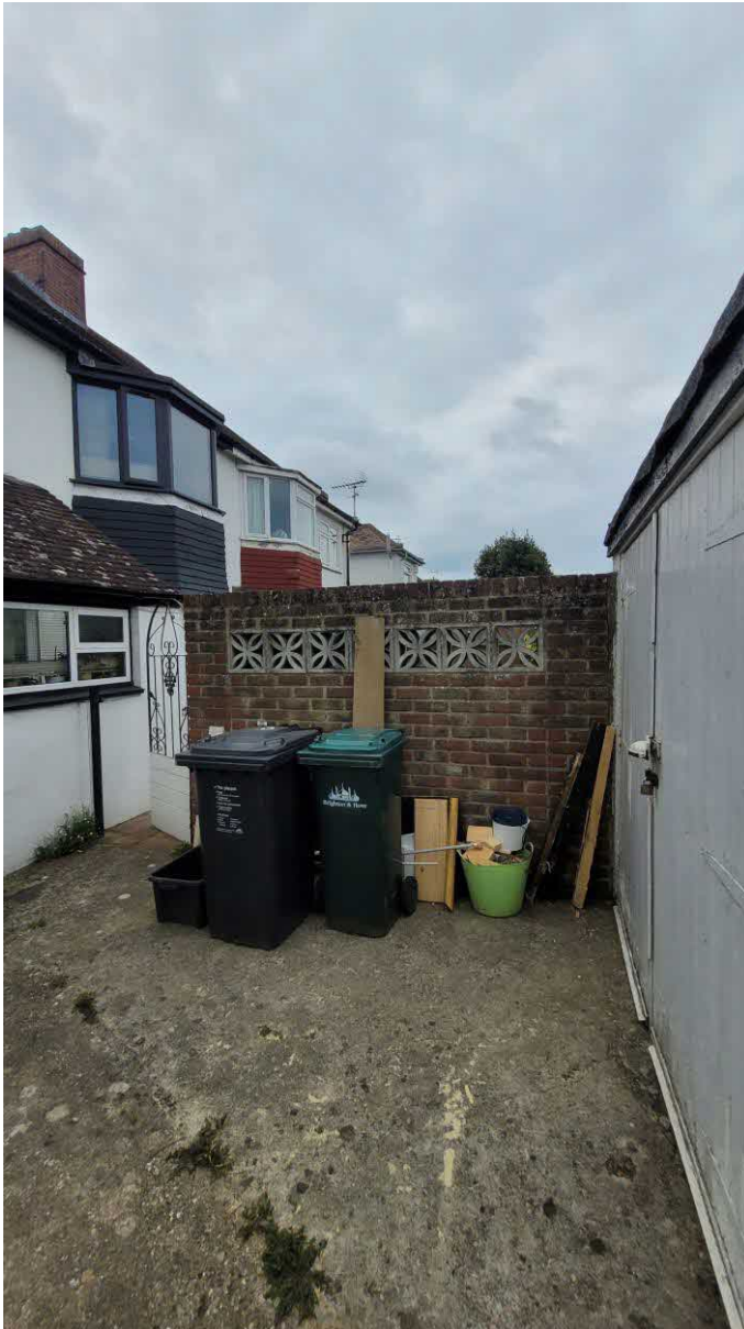
Side view of brick wall from shared driveway
