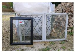
The photo above shows a sample of the proposed replacement metal framed window against the metal casement removed from the north gable. The leadwork can be made to match the diamond/diaper pattern of the existing window. The traditional detailing of the sample window would provide a replacement window that is consistent in materials and appearance whilst the double glazing would provide the benefit of improved thermal performance.
