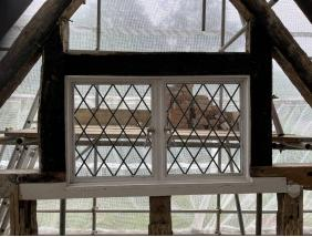
The photos above show an internal view and detail of the north gable attic window. This is a 20th century metal casement window with diamond pattern leadwork.
