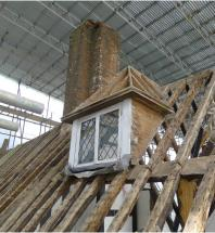
The photos above show the casement window to the west dormer, before repair works [left photo] and in the process of the repair works [roght photo]. This is the third window it is proposed to replace.
