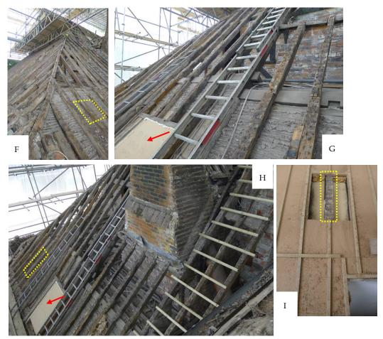
F: Detail of the lower north 'catslide' roof slope to the outshut; the yellow dashed rectangle shows the proposed location of the new roof light opening [ON-N-NEW-RL2] and the single common rafter that will need to be cut and trimmed to accommodate the roof light.
