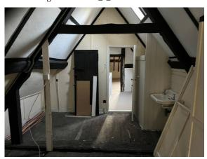
The proposed reinstatement of attic/second floor bathing facilities will be created by the provision of stud partition walls to replace lightweight soft-board walls to form the room.
