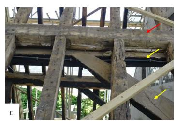
D: Detail from above of the east slope of the west range. Note the original purlin and brace [yellow arrows] and the later purlin [red arrow] showing a history of adaptation and alteration to the roof frame.
