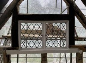
The photos above show an internal view and detail of the north gable attic window. This is a 20<sup>th</sup> century metal casement window with diamond pattern leadwork.
