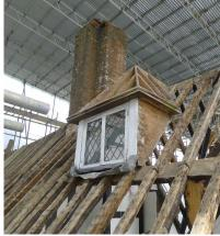
The photos above show the casement window to the west dormer, before repair works [left photo] and in the process of the repair works [roght photo]. This is the third window it is proposed to replace.
