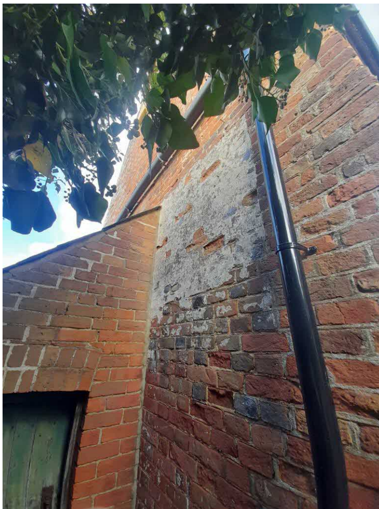
Photograph 7 Evidence of lime render/ limewash to adjoining wall
