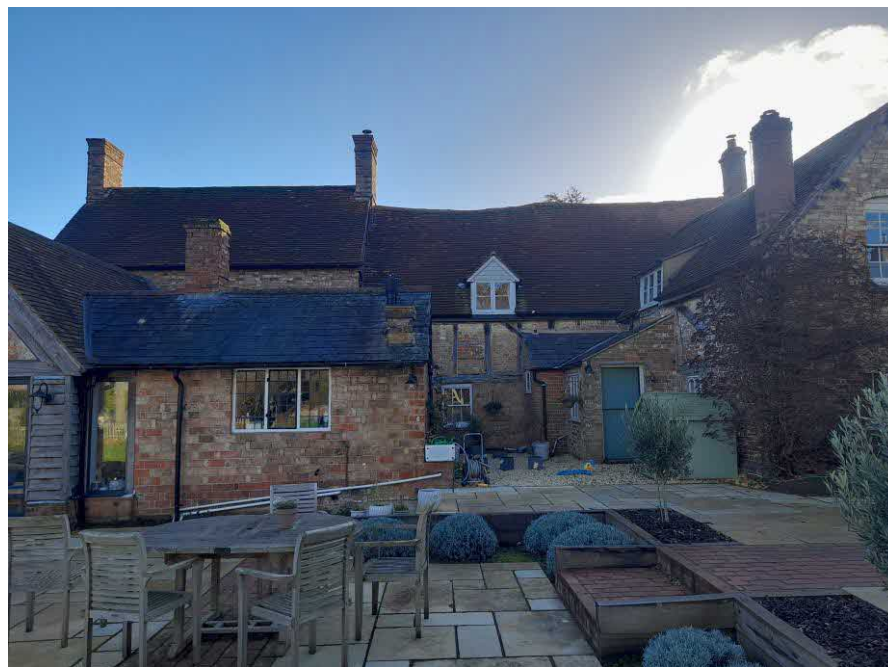
Photograph 19 Rear elevation of Mill Hook Farmhouse
