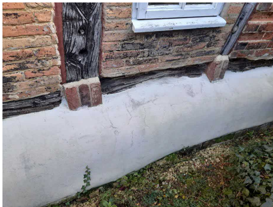
Photograph 4 Temporary repairs to shore up wall undertaken in 2021
