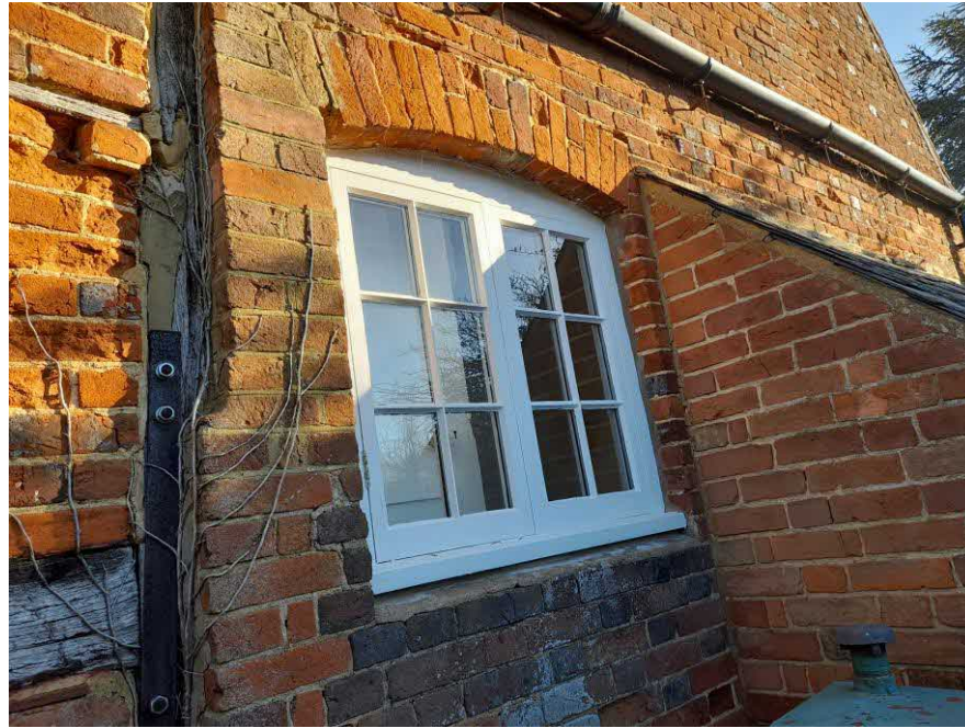
Photograph 12 Heritage slimline double glazed window replaced modern unit in 2021
