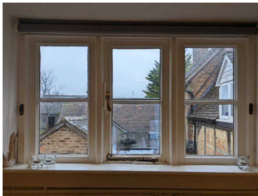
Photograph 13 Internal view of Bedroom window proposed for replacement
