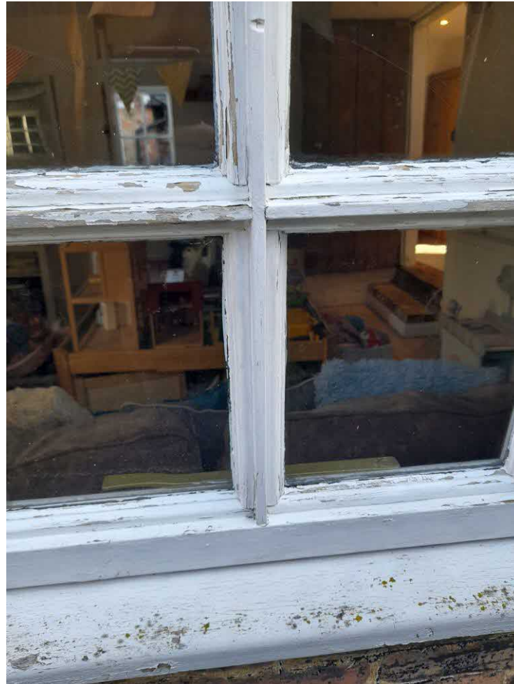
Photograph 10 Thick non-traditional glazing bars to right side window within South West facing timber frame panel
