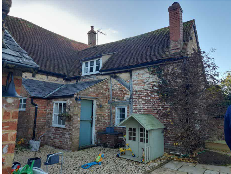
Photograph 8 Window to right of porch to be replaced
