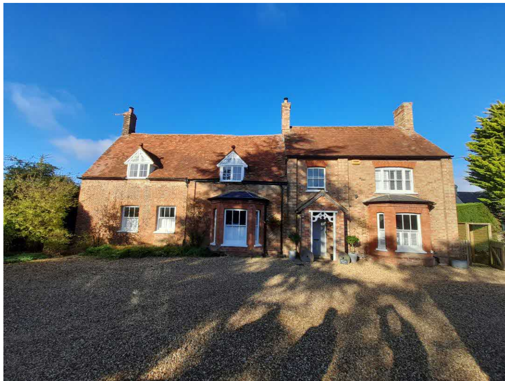
Photograph 1 Front elevation of Mill Hook Farmhouse
