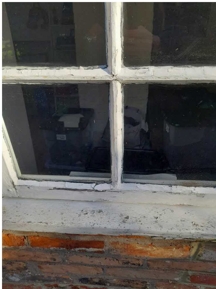
Photograph 11 Close up of modern glazing bars to left side window within South West facing timber frame panel
