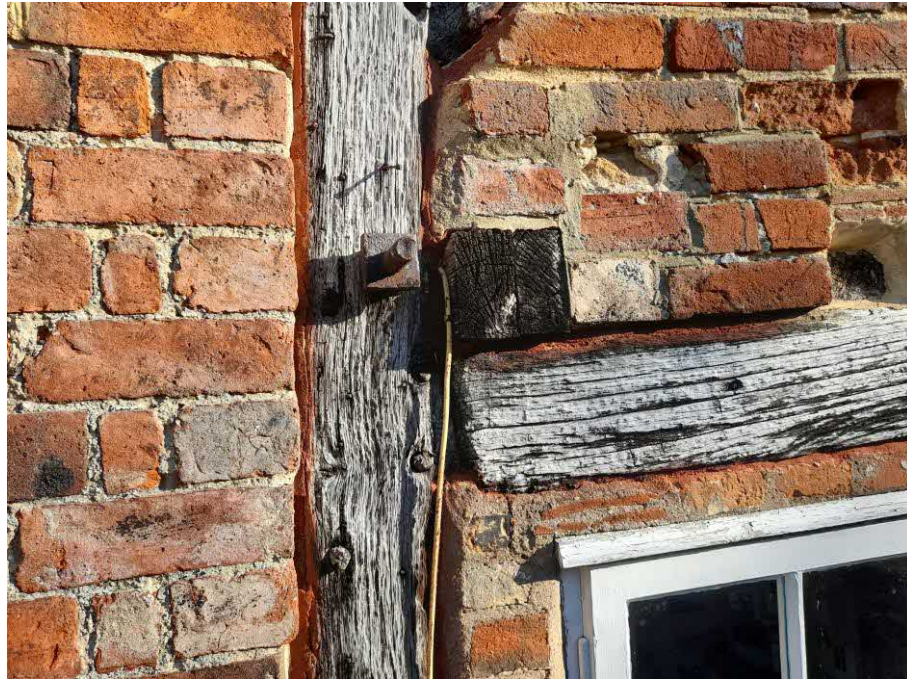
Photograph 6 Met al rod inserted through timber frame in 2021 to stabilize structure
