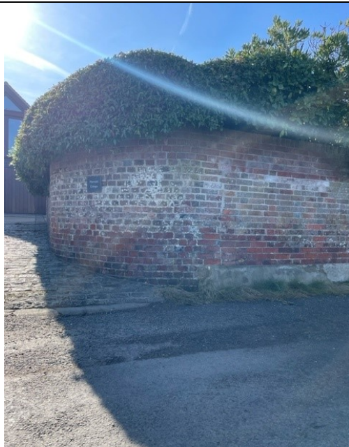
Image 1. View of the west end of the wall at the driveway return.
