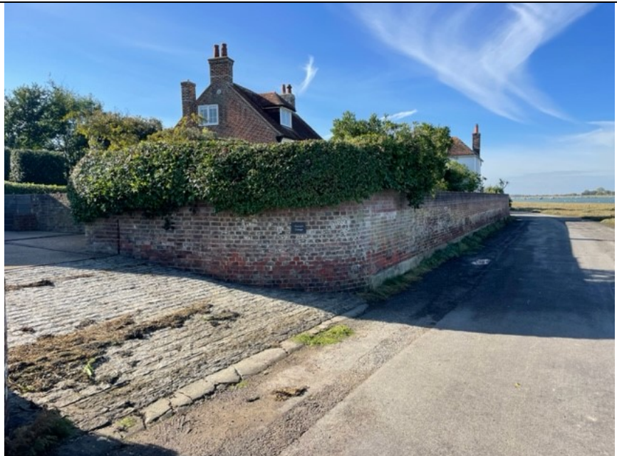
Image 2. Long view of the wall from the west.
