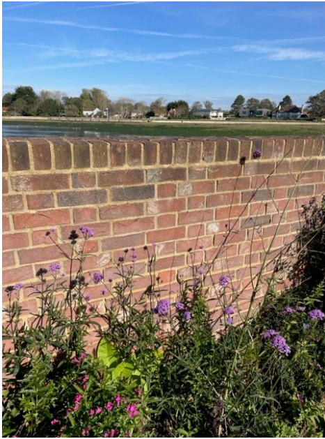
Image 1. View of the wall from the garden side.
