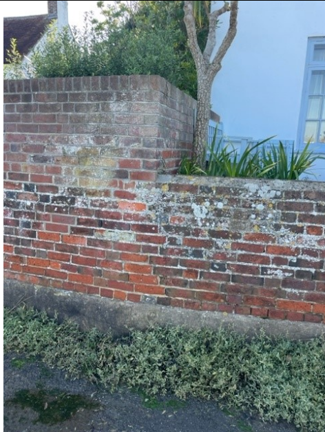
Image 5. Current difference in wall height at the East boundary. Proposal will remove the four brick courses under the coping course.
