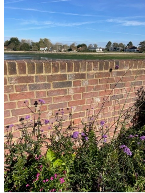
Image 6. View of the wall from the garden side.
