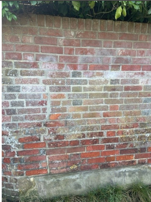
Image 3. Close up showing the variation in brick bonding (headers).
